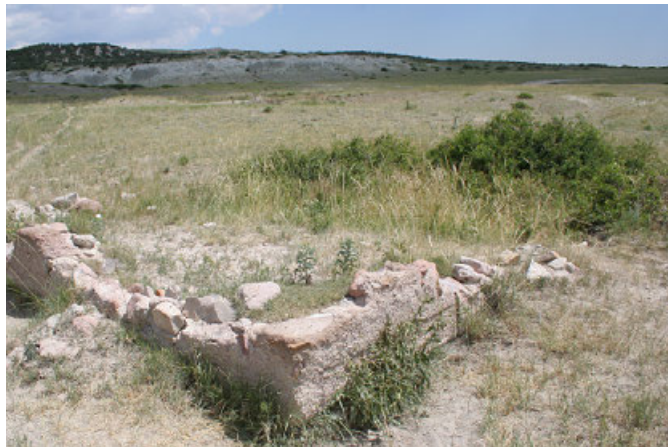
Southwest corner of Soapstone Springs School foundation. Construction of the foundation would have started here and proceeded counter clockwise; courtesy of Ken Jessen
