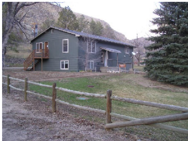
Ranger Office and Maintenance building
