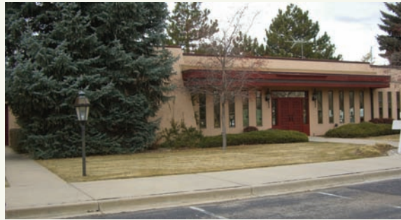
Pat Griffin Building – 303 W. Prospect Road
