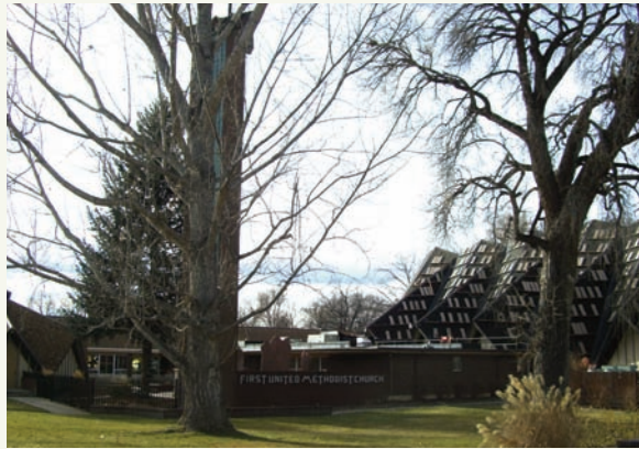
First United Methodist Church – 1005 Stover Street
