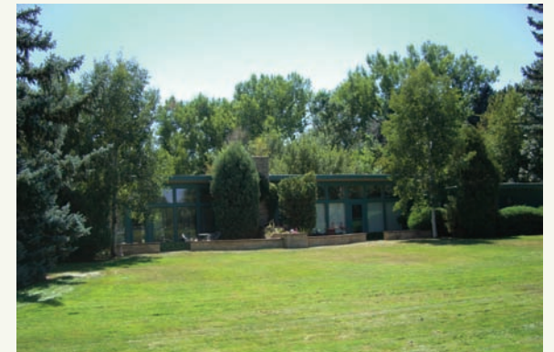
Davis-Gibson Duplex – 1607-1609 Mulberry Street
