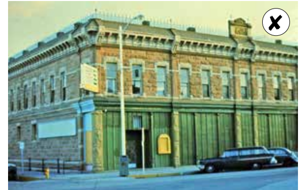
In 1979, wood paneling obscures historic storefronts.
