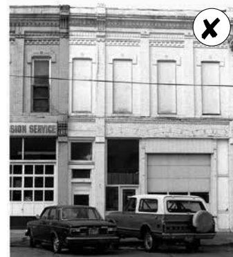
A close-up view of the storefront at 252 Linden, in 1980 shows the missing storefront.
