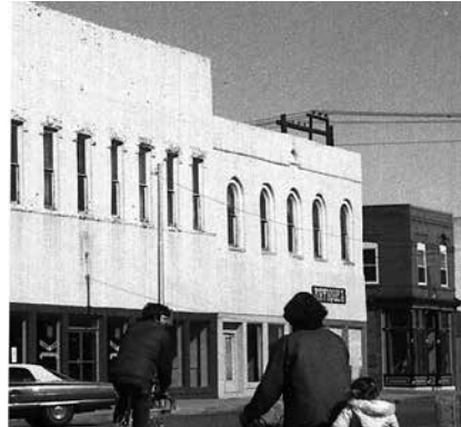
Before rehabilitation (ca. 1980)
