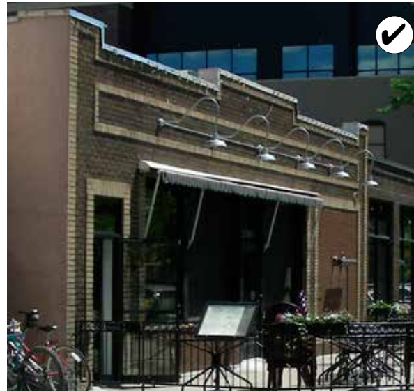
Early Twentieth - Century Commercial, single storefront.
