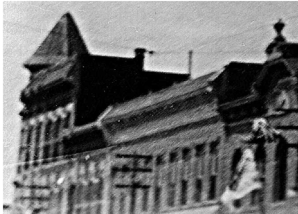
Use historic photos as a source for reconstructing a missing detail.
