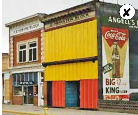
In 1980, metal cladding obscures most of the key character-defining features of the building front.
