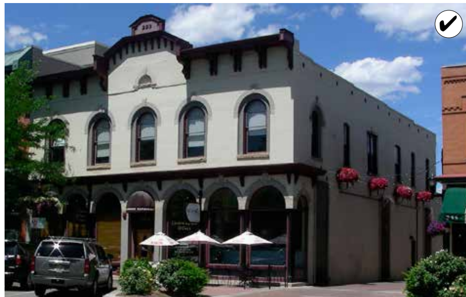
The rehabilitated Reed and Dauth building, 223 Linden Street (2013)
