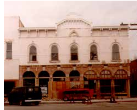
During rehabilitation (ca. 1982)
