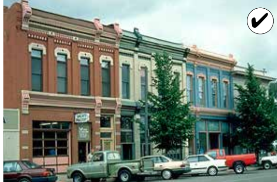
After rehabilitation in the mid-1980s, many storefronts have been reconstructed. Architectural details are highlighted with contrasting color schemes. The left-most storefront remains altered, but other features on this facade have been preserved.
