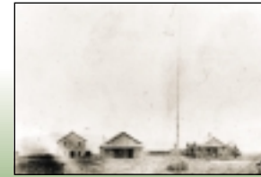
Poudre gristmill & various buildings, c1865
