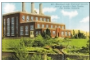
Municipal Light Plant, c.
