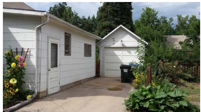
Figure 4-13: Small garage behind 106 S. Loomis, accessed from street (Carly-Ann Anderson, 2014).
