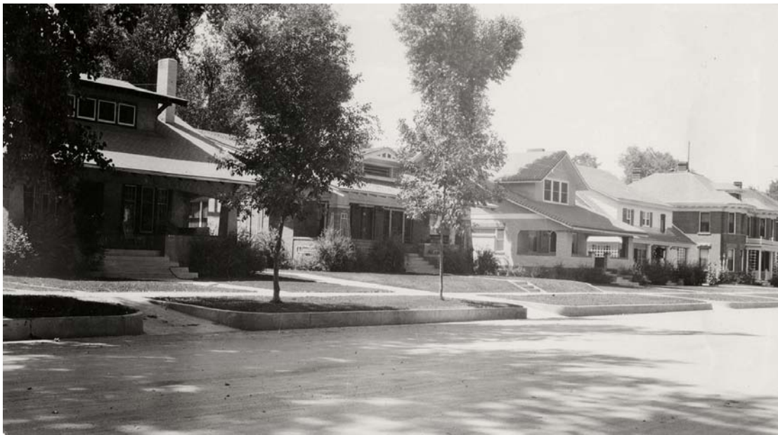
Figure 4-10: West Mountain Avenue in 1924, showing Craftsman, Dutch Colonial and American Foursquare houses (University Historic Photograph Collection, Colorado State University, Archives and Special Collections).
