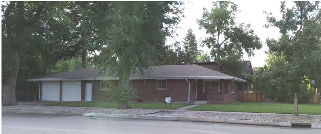
Figure 8-32: Ranch-style home at 231 S. Whitcomb St., built in 1964 – the last house built in the Loomis Addition during the historic period (Carly-Ann Anderson, 2014).
