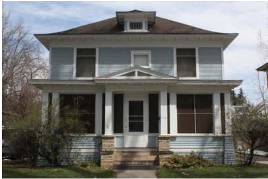
Figure 8-1: American Foursquare house, 714 W. Mountain Ave. (Meg Dunn, 2013).
