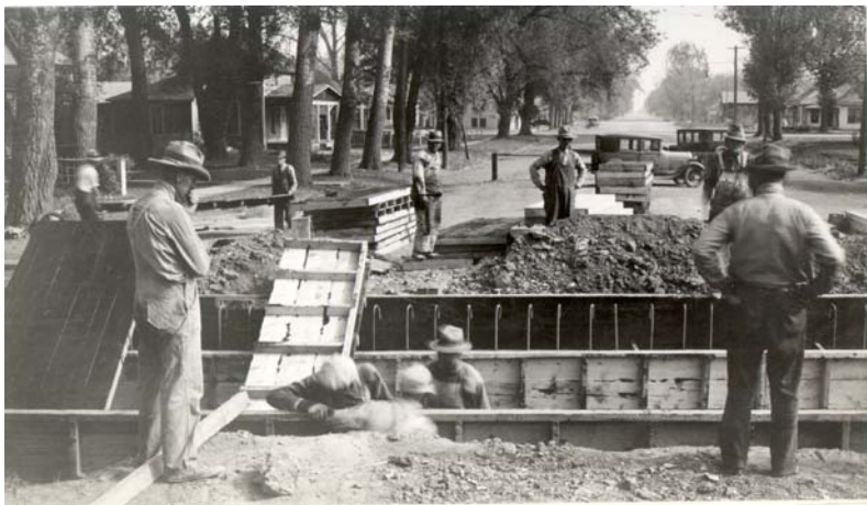
Figure 5-3: Covering the Town Ditch, 1933 (Local History Archive H20073).
