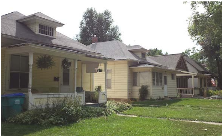
Figure 6-7: 800 block of West Mountain Avenue (Carly-Ann Anderson, 2014).
