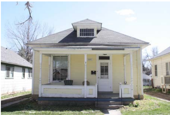
Figure 8-11: House at 805 W. Mountain Ave., built by Morrison & Madden and Roys & Hampton (Meg Dunn, 2013).
