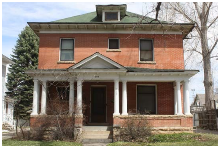
Figure 7-10: Dr. De Armond House, 708 West Mountain Ave. (Meg Dunn, 2013).
