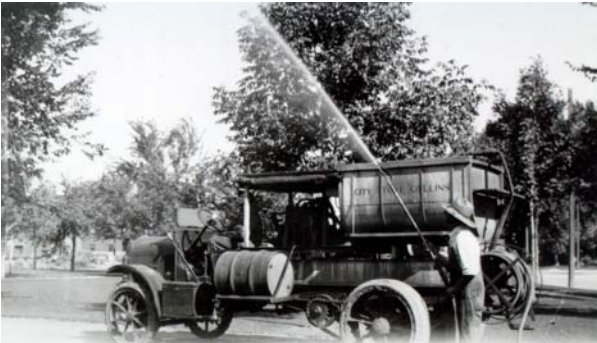
Figure 3-4: Bill Frye spraying city streets to keep down dust, c. 1927 (Local History Archive H14858).
