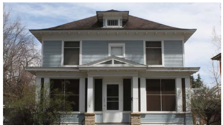
Figure 8-20: American Foursquare house at 714 W. Mountain Ave. has simple detailing and slightly flared roof eaves (Meg Dunn, 2013).
