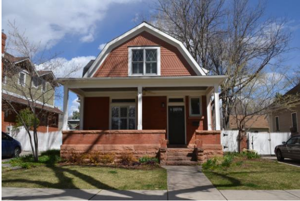
Figure 5-22: 722 W, Mountain. Windows on façade have been replaced, but are consistent with overall design and the rest of the house retains good integrity; contributing (Mary Humstone, 2016)
