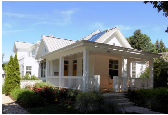
Figure 5-18: 119 N. Loomis. Two-story addition at rear of house is larger than original portion of house and clearly visible from public ROW; non-contributing (Luke Anderson, 2016)
