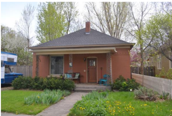
Figure 5-17: 611 Laporte. Porch altered during period of significance; contributing (Mary Humstone, 2016)
