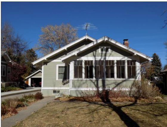
Figure 5-21: 712 W. Oak. Siding replaced with same material and profile as original; contributing (Luke Anderson, 2016)
