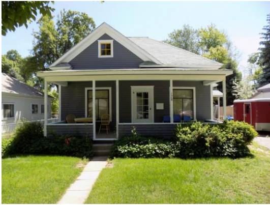
Figure 5-19: 128 N. Loomis. Small, one-story rear addition not easily visible from public ROW; contributing (Luke Anderson, 2016)
