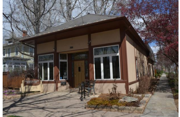
Figure 5-23: 700 W. Mountain. Windows and openings have been altered and the building's original false-front façade has been altered; non-contributing (Mary Humstone, 2016)
