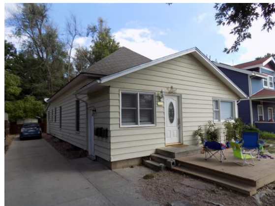
Figure 5-20: 608 W. Magnolia. Original wood siding was replaced with wide-lap synthetic siding, changing the character of the house; non-contributing (Luke Anderson, 2016)
