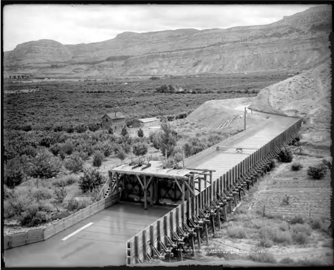
Figure 18. Large wooden flume on Orchard Mesa Canal, Mesa County. Photographed by Louis Charles McClure, c. 1911. The flume crosses a natural drainage and protects the canal from washing out.
