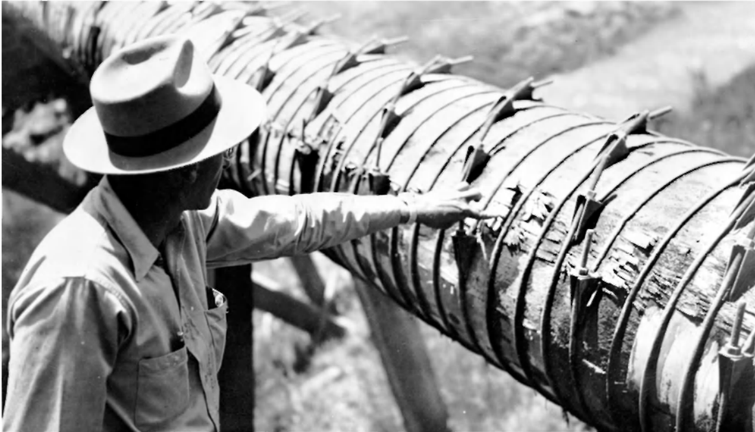
Figure 19. Wood-stave siphon pipe on the Montezuma Valley irrigation system, constructed c. 1885, photographed in 1951.
