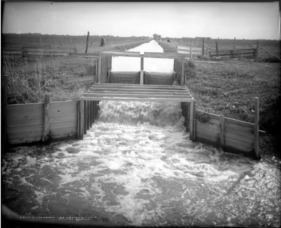
Figure 22. Simple wooden drop structure on a ditch on the eastern plains. Photographed c. 1900-1920 by Louis Charles McClure.
