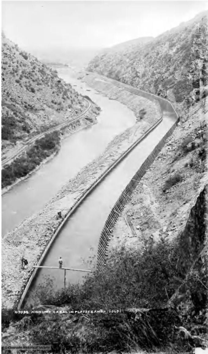
Figure 5. High Line Canal in Platte Canyon, circa 1883. Photographer: William Henry Jackson. A wooden bench flume carries the canal on a shelf blasted into the side of the canyon.
