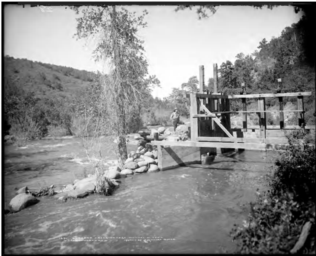
Figure 13. Headgate for Mutual Ditch on Buzzard Creek in Plateau Valley, Mesa County. Photographed by Louis Charles McClure c. 1911. Headgate is wooden with steel control mechanisms. Diversion works consist of a temporary rubble dam in the stream.
