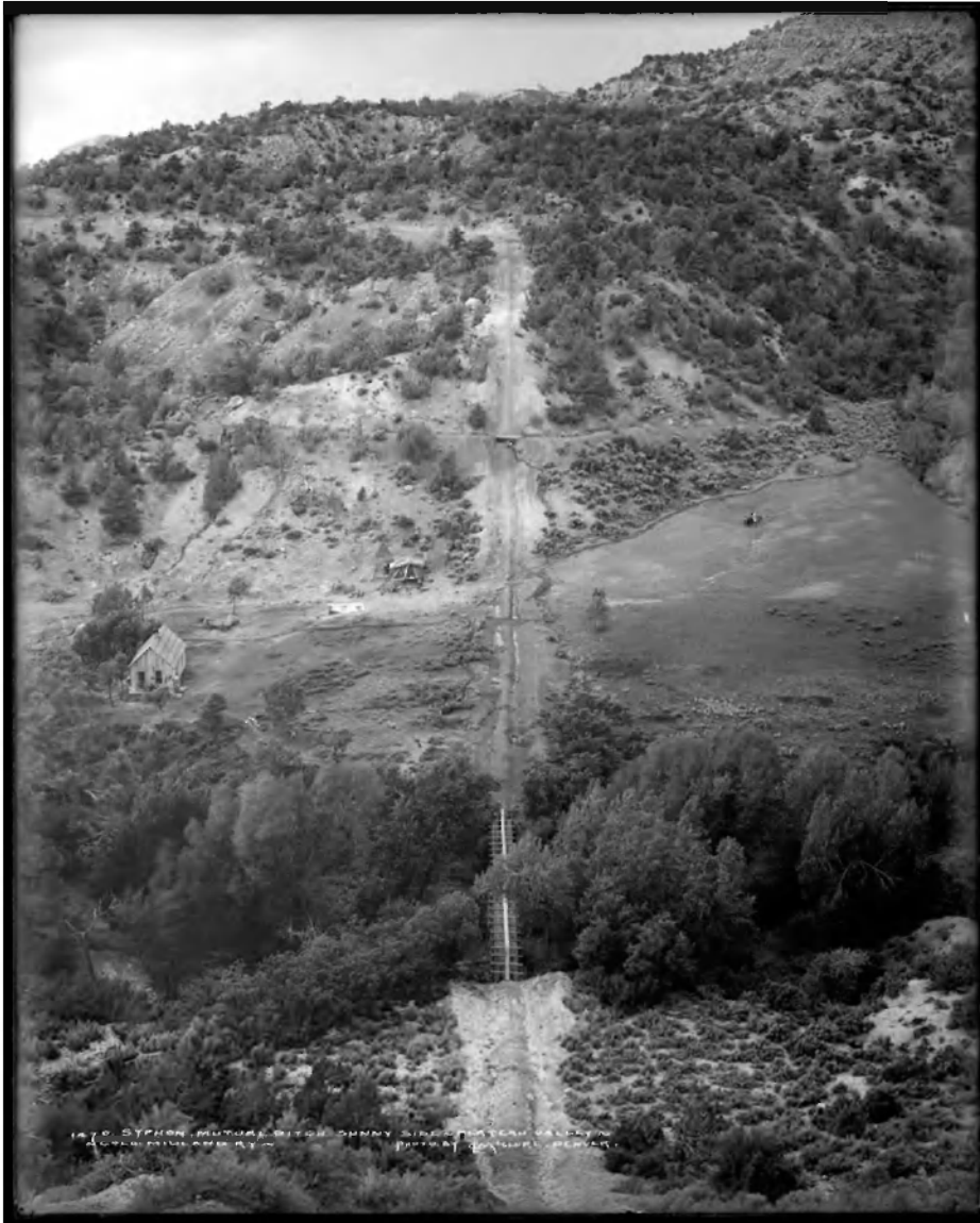
Figure 20. Mutual Ditch siphon, Sunnyside, in Plateau Valley, Mesa County. Photographed by Louis Charles McClure, c. 1911. A lower ditch crosses the siphon on a wooden flume, feeding a lateral that crosses the siphon again, on an earthen berm.
