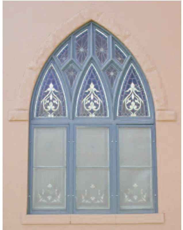
Figure 14. Detail of an exquisite stained-glass, gothic-arched window, on the east elevation of the German Evangelical Congregational Church. Churches are the German-Russian community's most visible architectural contributions to Fort Collins. (Photo by the author.)
