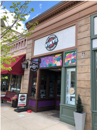
120 S. College Avenue – Mossman Building
