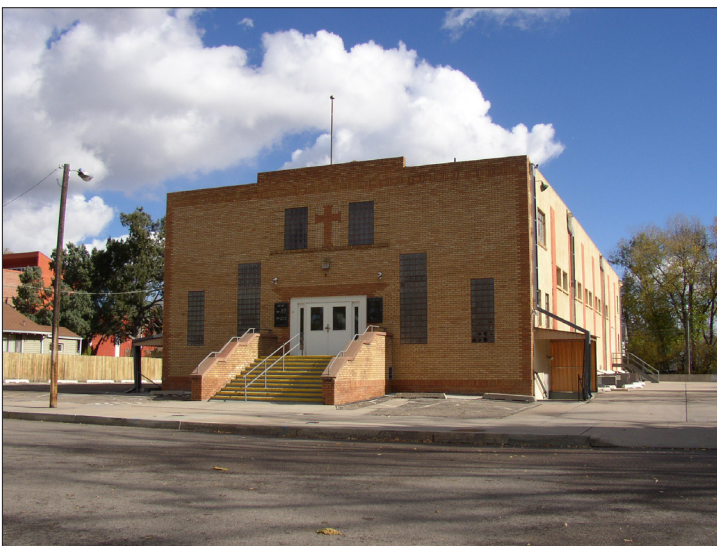
Figure 2. Holy Family parish hall, 324 N. Whitcomb Street
