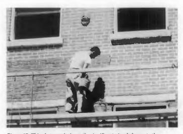
Figure 17. This photograph shows the significant visual change to the character of this historic brick building that has resulted from improper repointing procedures and a noticeably increased thickness of the mortar joints. Photo: Lee H. Nelson, FAIA.
