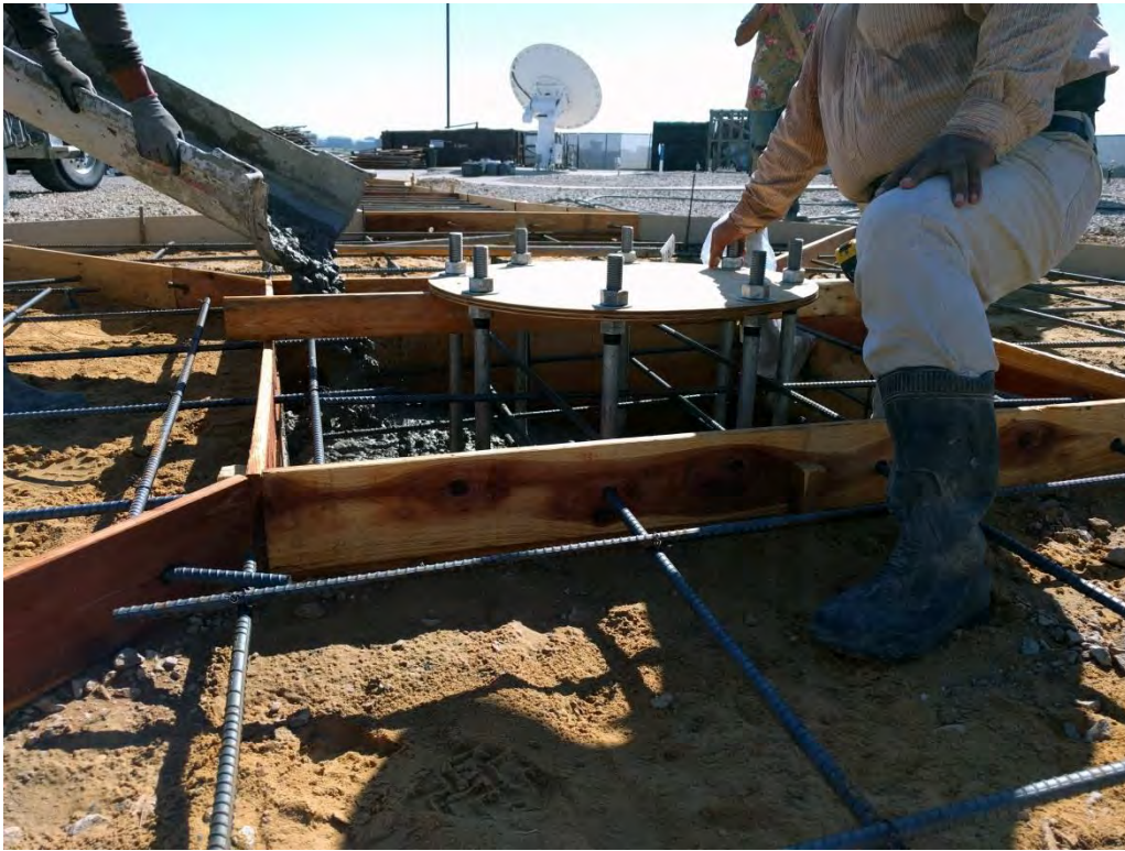
Figure 21 - Concrete Foundation for Ground Mounted Positioner (Example Only)
