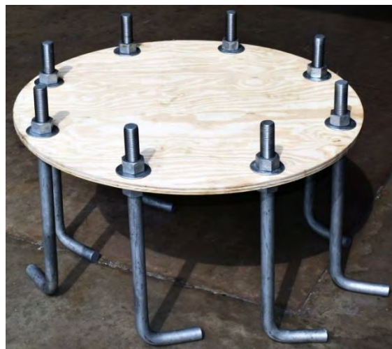
Figure 20 - Plywood Template with Studs Prior to Installation in Wet Concrete
