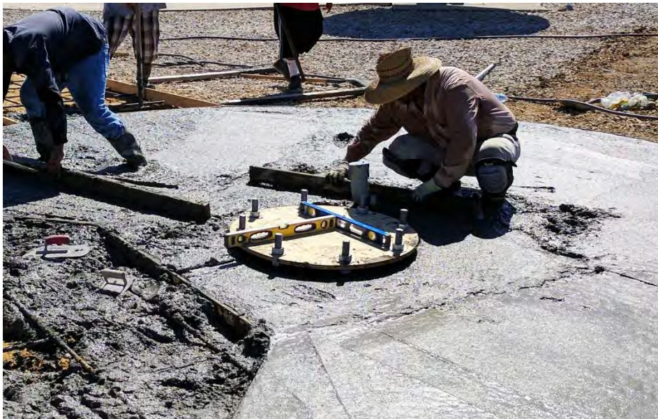
Figure 22 - Installing Studs in Wet Concrete Using the Plywood Template
