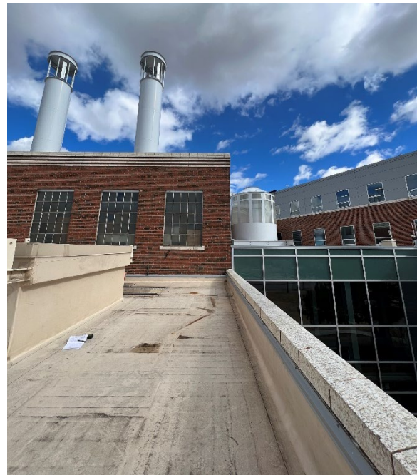
Fig 6. Roof image at construction zone
