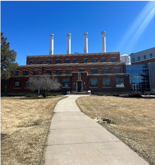
Fig 5. Sidewalk View of Powerhouse West
