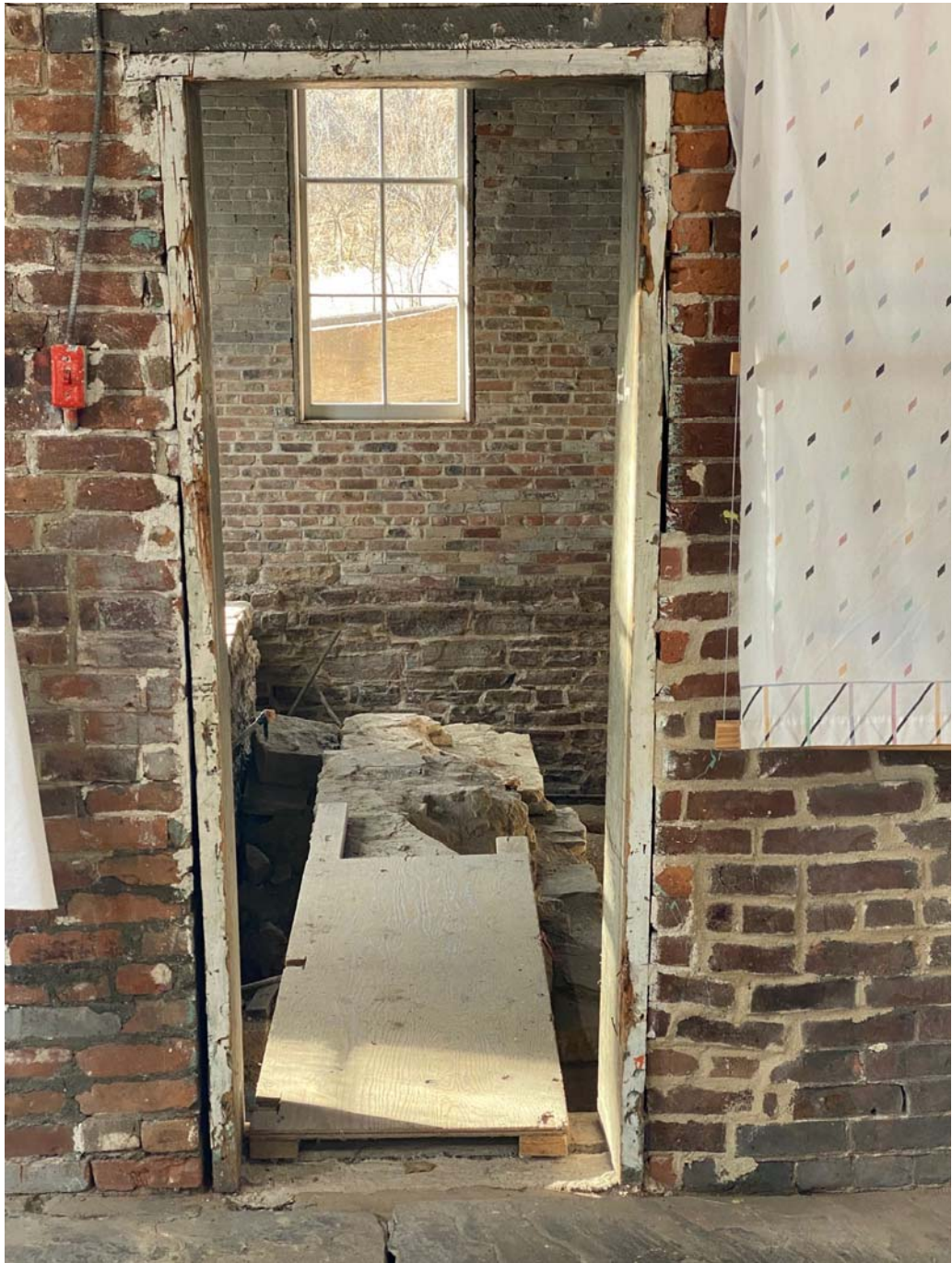
Picture 5, Existing Pump Room Doorway
