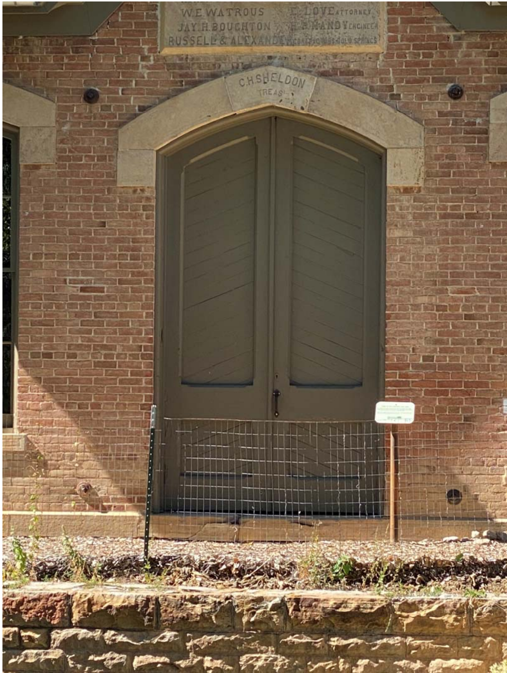
Picture 3, Existing Front Door & Fence
