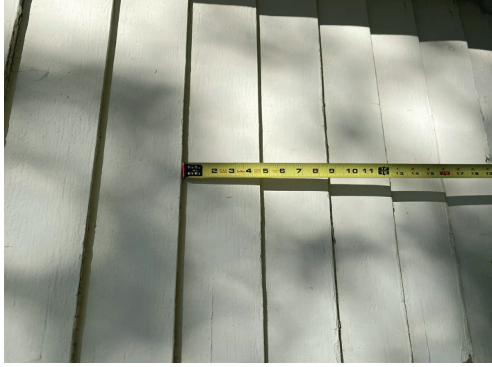
North Side lap siding, 5" exposure
