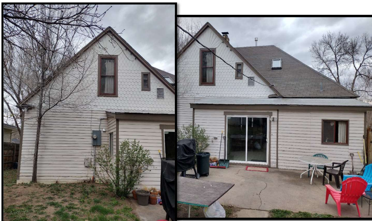
Figure 3: Rear of House
