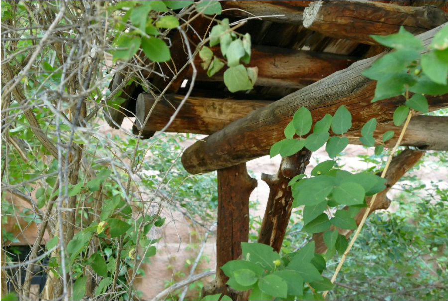
Wishing Well Structure Northwest corner – outside
