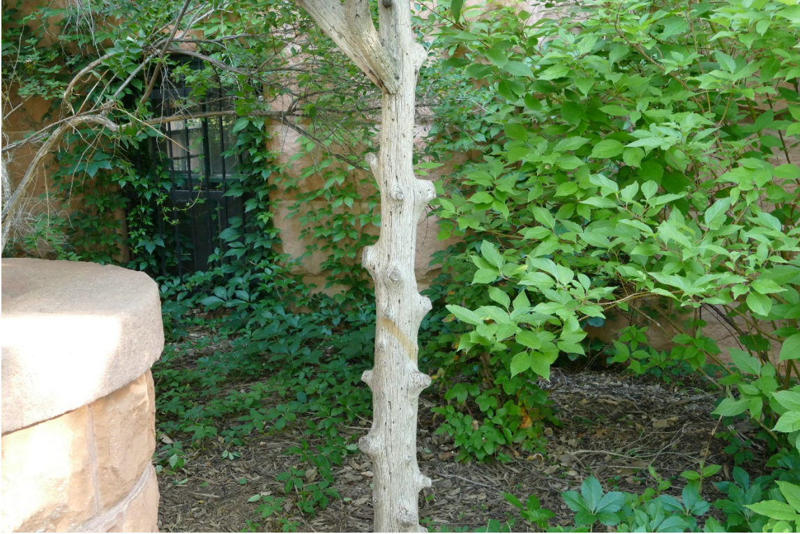
Wishing Well Structure Northeast Post
