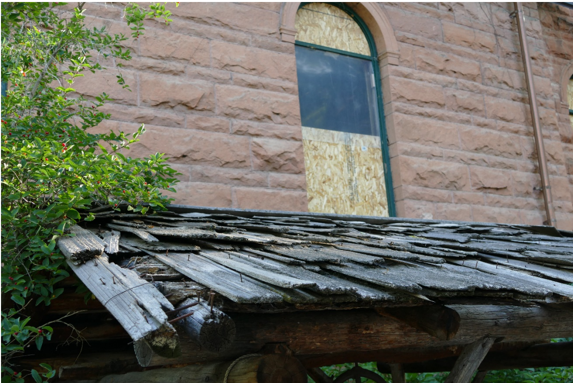
Wishing Well Structure roof
