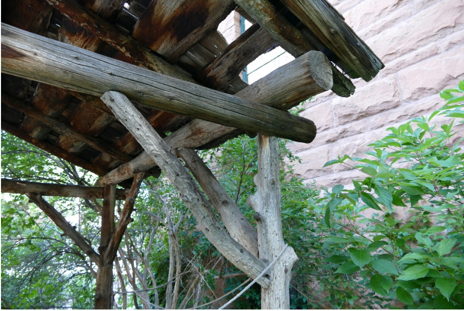
Wishing Well Structure Northeast corner - outside
