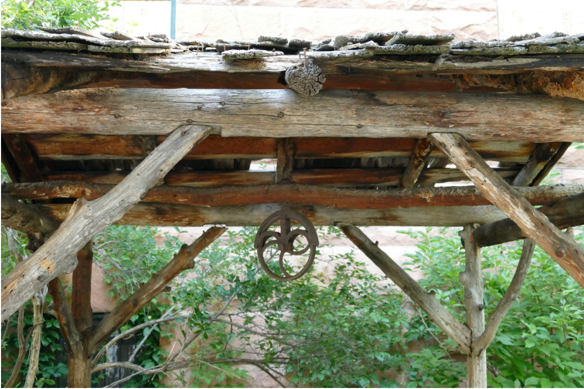
Wishing Well Structure South view
