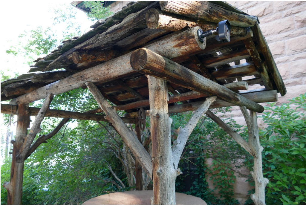
Wishing Well Structure Southeast corner – outside.
