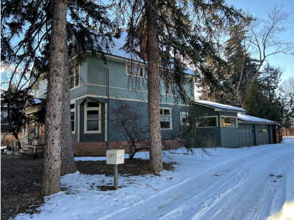
North elevation, looking southwest
