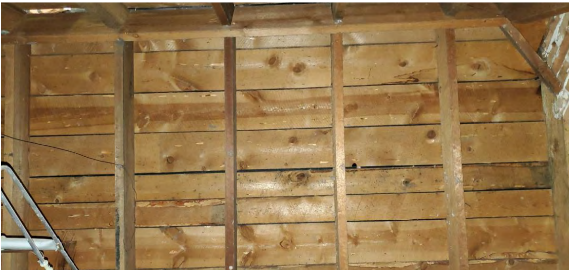
Figure 3. View looking up of existing roof framing and decking from attic interior.
