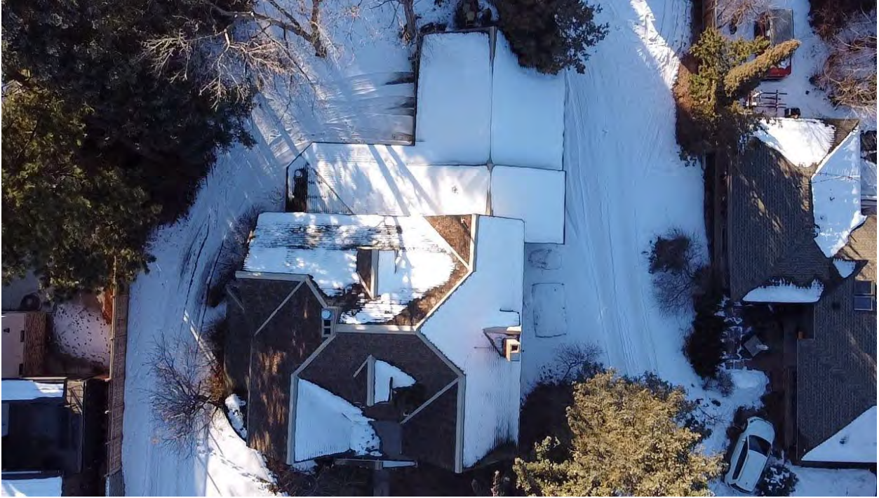
Aerial, showing roof
