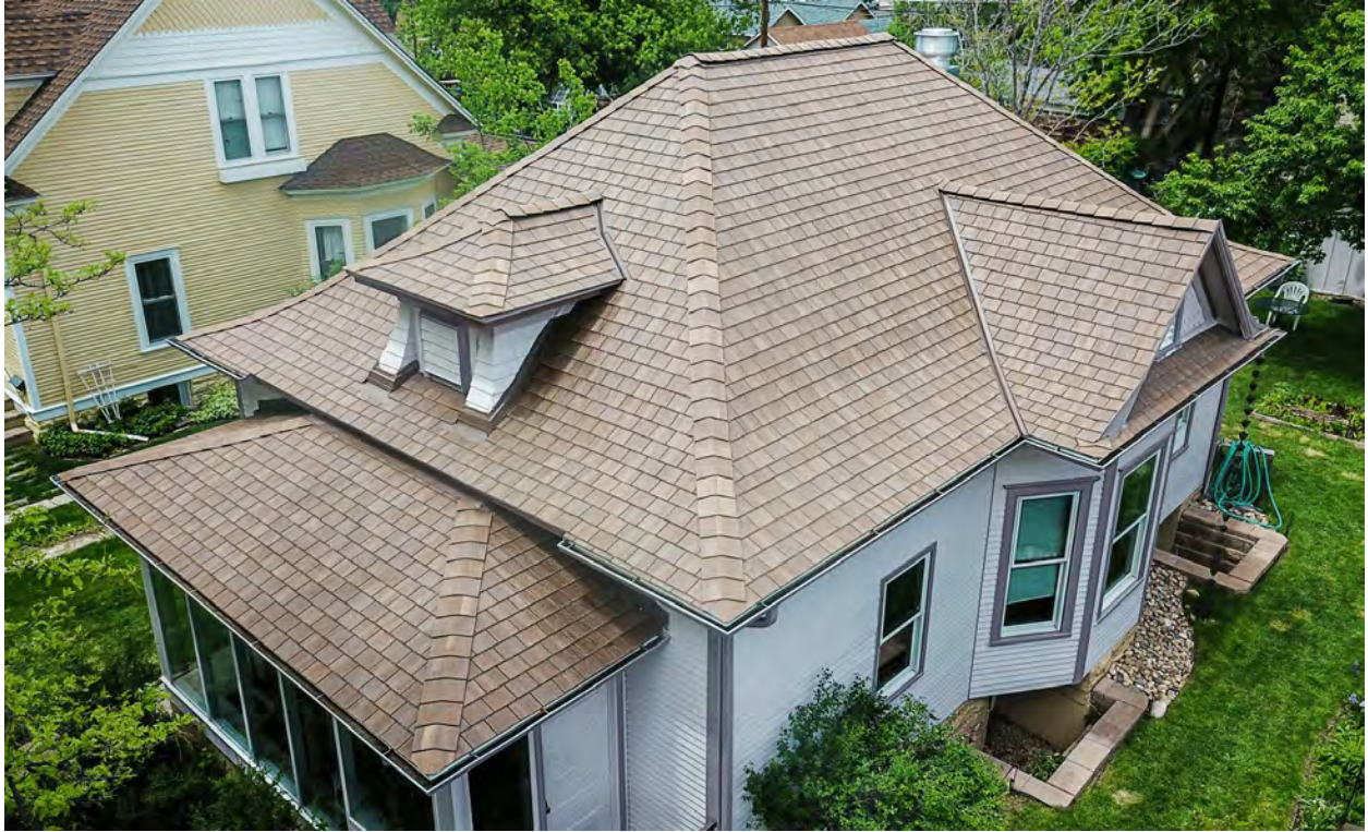
220 E. Elizabeth, F-wave installation
