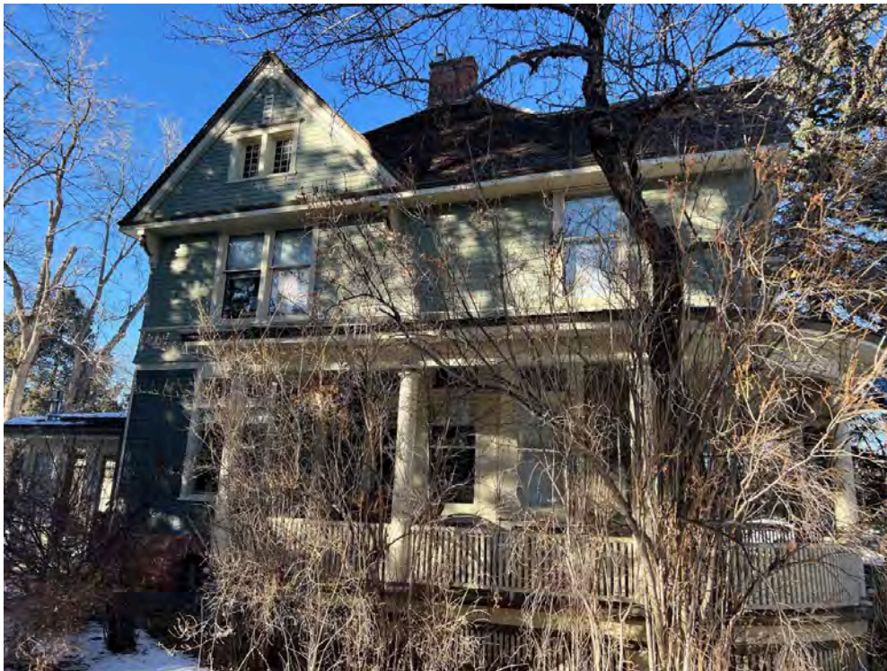
South elevation, looking north
