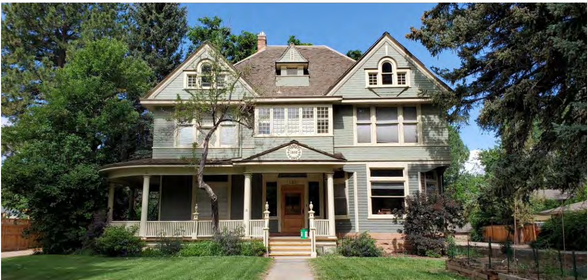
Figure 1. Overall view of residence at 113 N Sherwood Street.
