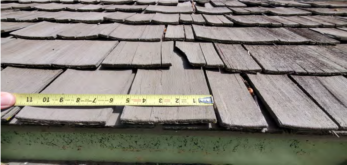
Figure 2. Close-up view of existing wood shingles.
