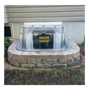
I called the manufacturer, Shape, and the man I spoke to said that this style should work for an outswing casement egress window. He also said that they normally have clips to attach to metal window wells, but they make adapter kits for attachment to timber window wells too. Although they don't have a weight-rating on their technical sheet, the employee was confident that it could support 250 lbs because of the polycarbonate material.
