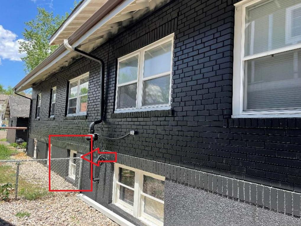
IN CASES WHERE THE NEW EGRESS WINDOW R.O. IS LESS THAN OR EQUAL TO THE EXISTING WINDOW WIDTH, THE EXISTING HEADER/LINTEL IS SUFFICIENT TO SUPPORT THE MAXIMUM DESIGN LOADS IMPOSED. NO ADDITIONAL SUPPORT REQUIRED. LEAVE SIDES AND TOP OF EXISTING METAL WINDOW
