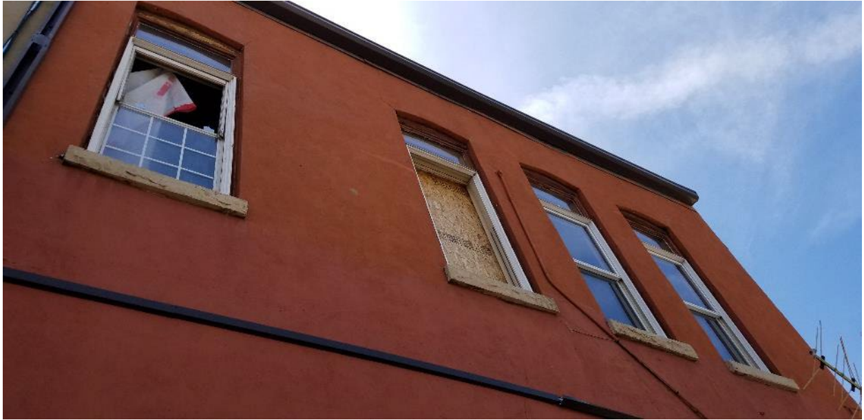
Upper floor on rear elevation above the garage entry.
