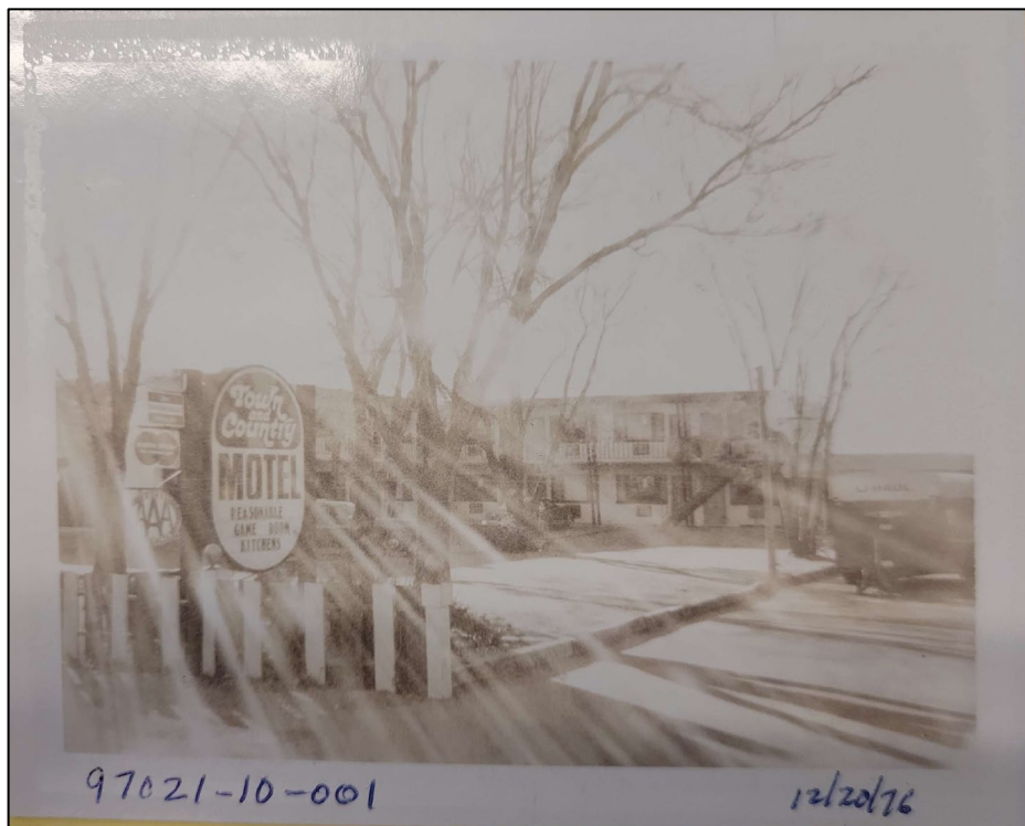
Figure 10: Feature 2, Larimer County Tax Assessor photograph, 1976. Image on-file with Fort Collins Museum of Discovery.
