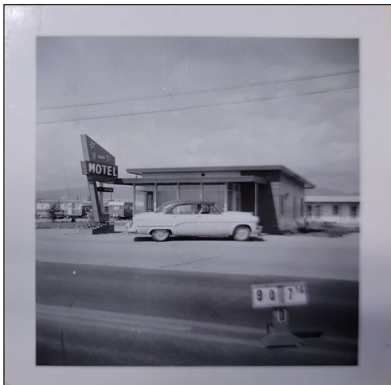
Figure 4: Feature 1, Larimer County Tax Assessor photograph, 1956. Image on-file with Fort Collins Museum of Discovery.
