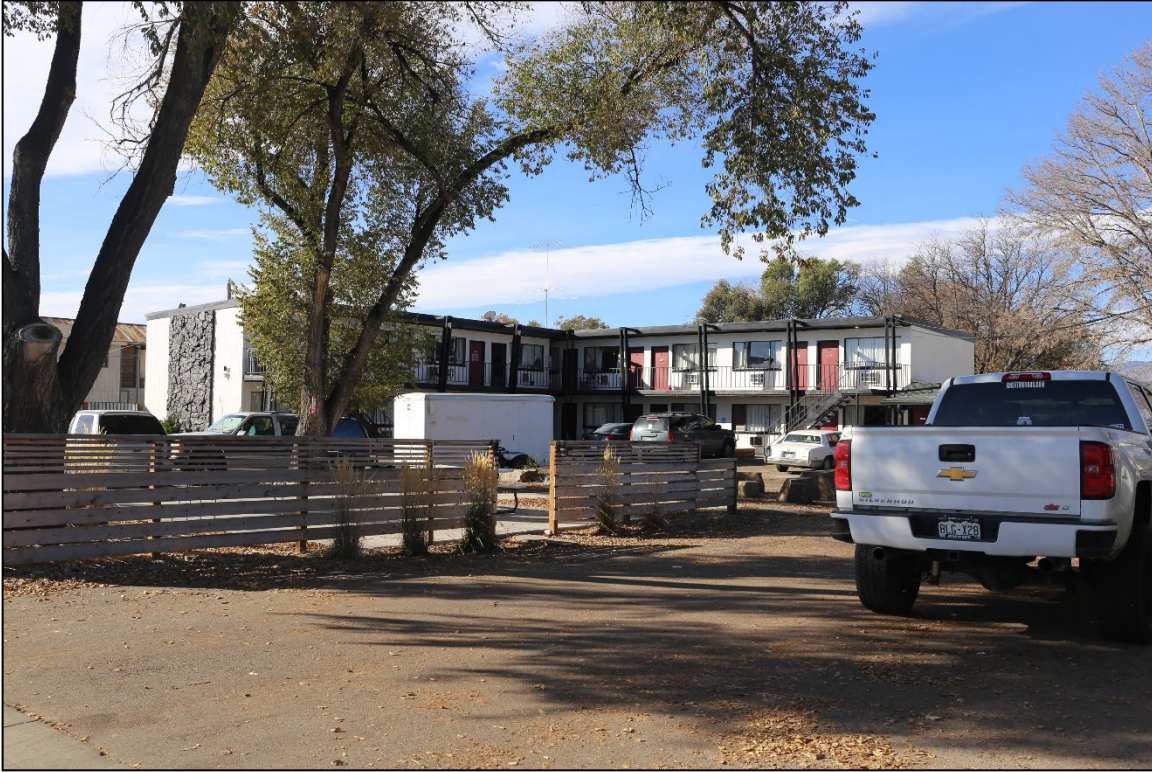
Figure 14: Feature 2, east and north elevations, view southwest (Image #7492, R. Shields, 11/2/2023).
