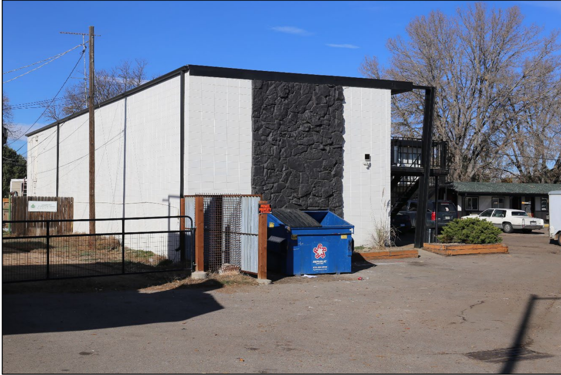
Figure 16: Feature 2, south and east elevations, view northwest. Note Feature 3 in background at right. (Image #7485, R. Shields, 11/2/2023).
