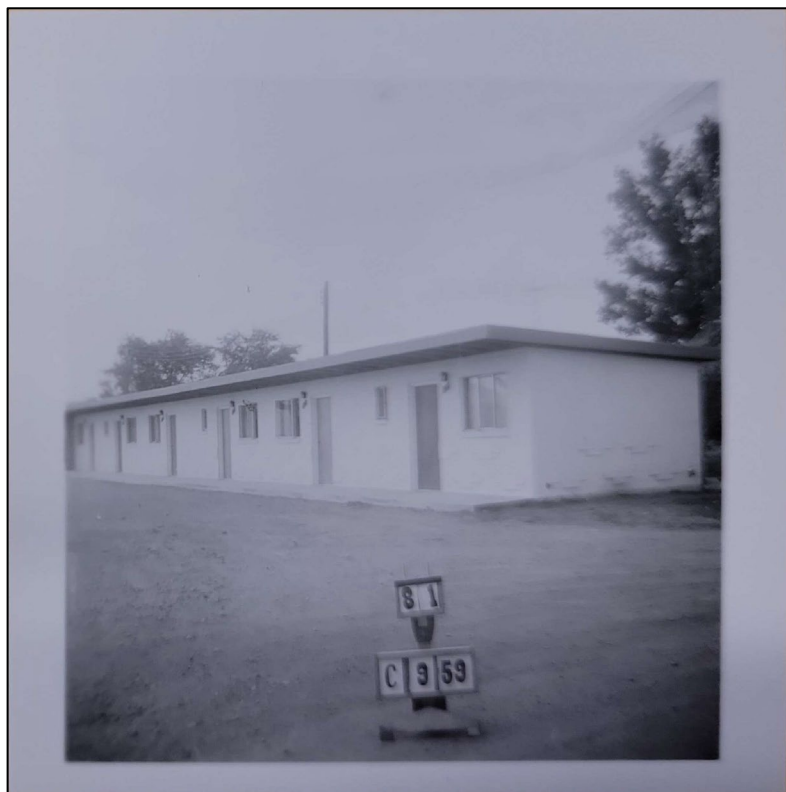
Figure 5: Feature 5, Larimer County Tax Assessor photograph, 1959. Image on-file with Fort Collins Museum of Discovery.
