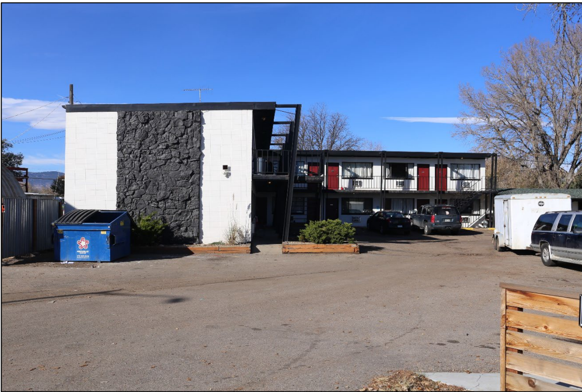
Figure 15: Feature 2, east elevations, view west (Image #7487, R. Shields, 11/2/2023).
