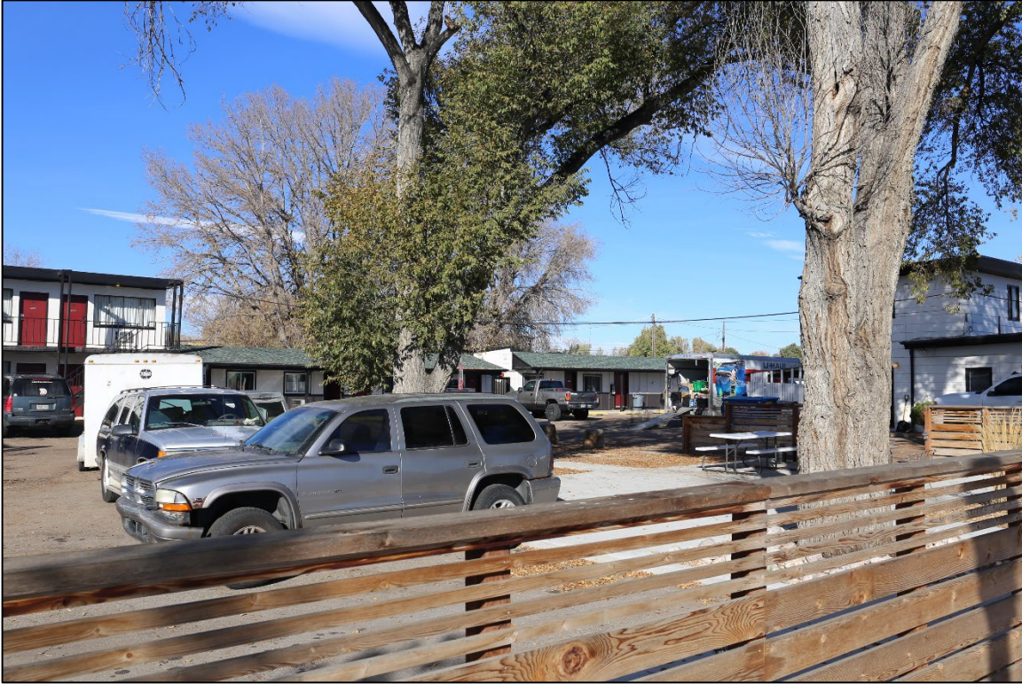
Figure 18: Feature 4 at center right, east elevation, view northwest. Note Features 2 and 3 at left and Feature 1 at right. (Image #7488, R. Shields, 11/2/2023).
