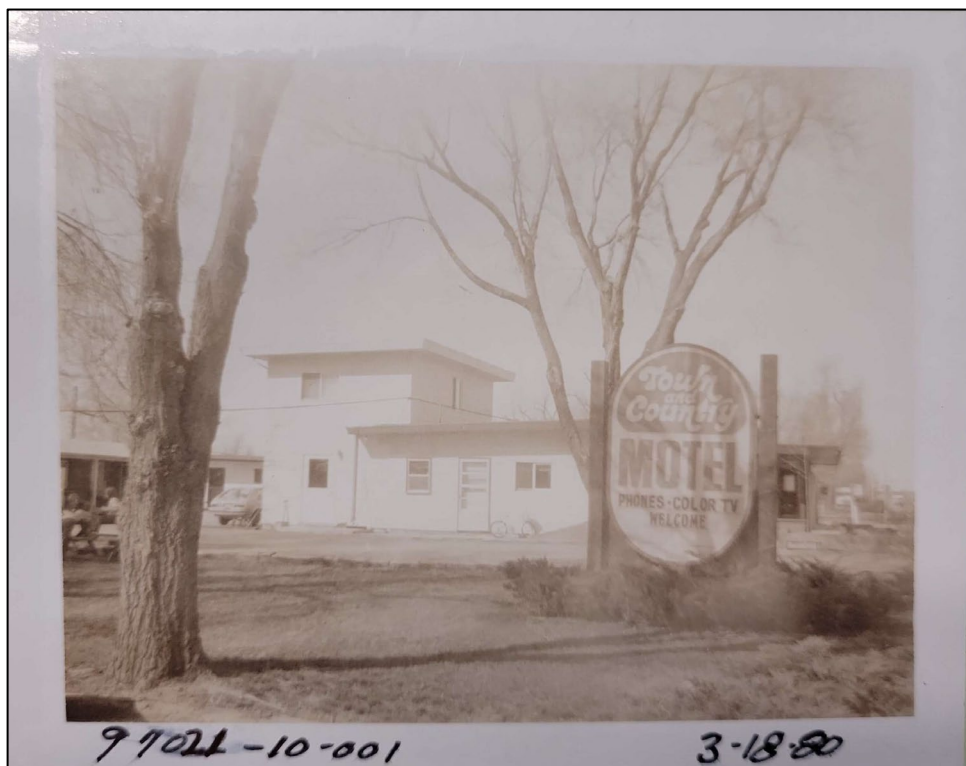
Figure 11: Feature 1, Larimer County Tax Assessor photograph, 1980. Image on-file with Fort Collins Museum of Discovery.
