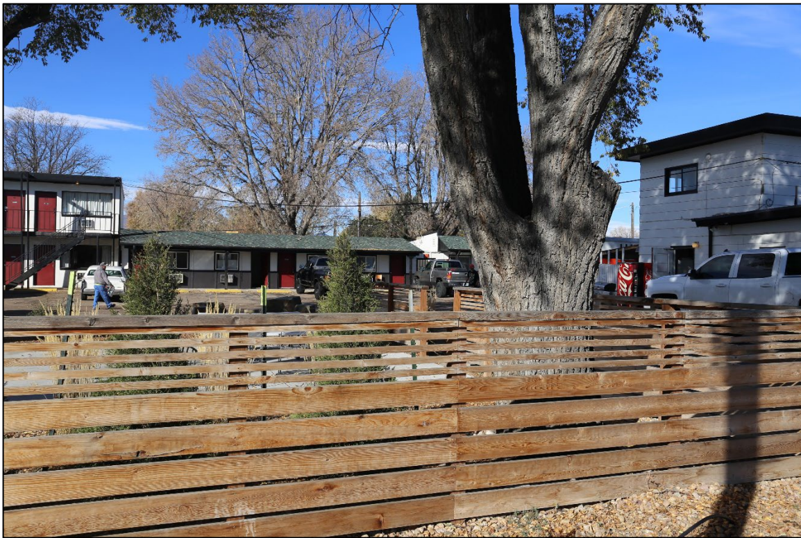
Figure 17: Feature 3 at center, east elevation, view northwest. Note Feature 2 at left, Feature 4 at center right, and Feature 1 at right. (Image #7491, R. Shields, 11/2/2023).
