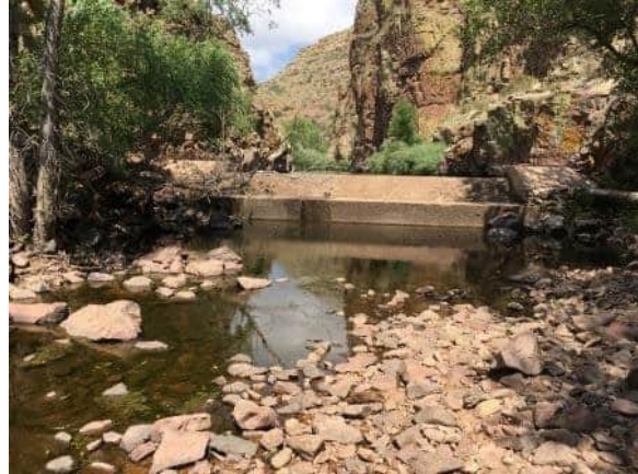
Figure 5-2. Calloway Diversion Structure
