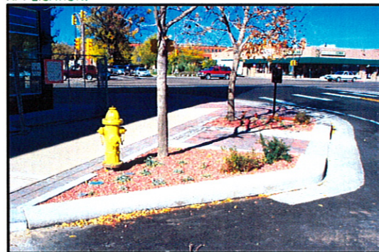
EXISTING OLD TOWN BULB-OUT SHOWING PAVING PATTERNS AND PLANTING AREAS.
