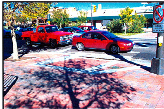
EXISTING OLD TOWN CORNER DETAIL SHOWING PAVING PATTERNS, TREE GRATE AND CONCRETE WORK.
