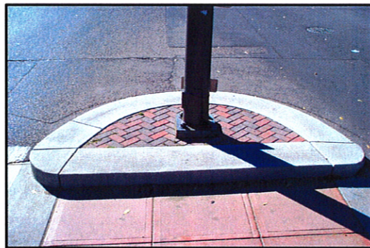
EXISTING OLD TOWN MEDIAN NOSE WITH 8'X8' CONCRETE PAVERS
