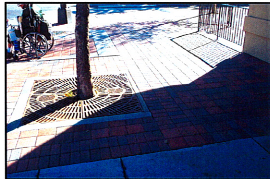
EXISTING OLD TOWN CORNER DETAIL SHOWING PAVING PATTERNS, TREE GRATE, AND TRANSITION TO CONCRETE SIDEWALK.
