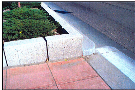
EXISTING OLD TOWN PEDESTRIAN REFUGE IN MEDIAN
