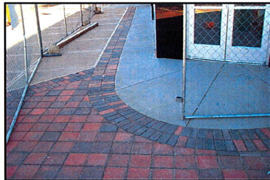
EXISTING OLD TOWN CORNER DETAIL SHOWING PAVING PATTERNS AND CONCRETE WORK FOR RADIAL APPLICATION.
