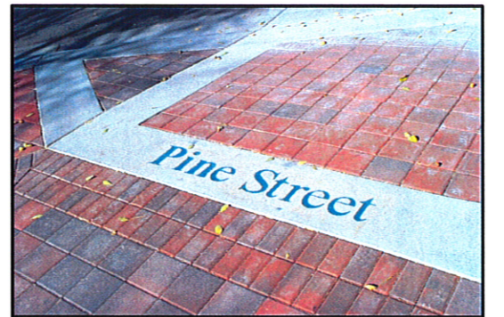
EXISTING OLD TOWN RAMP SHOWING PAVING PATTERN, CONCRETE WORK AND STREET NAME
