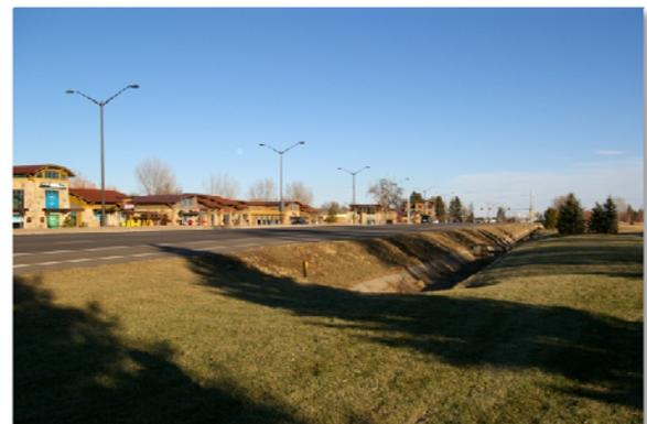
*This photo illustrates large setback adjacent to Harmony Road and an example of a concrete lined ditch that separates the roadway from the corridor land uses.*
