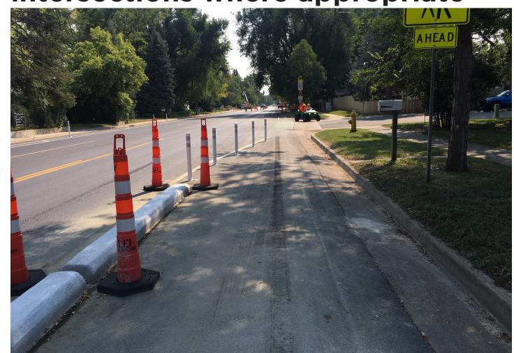
Adjust parking curb stops around lake to increase bike lane width and prevent vehicle overhang
