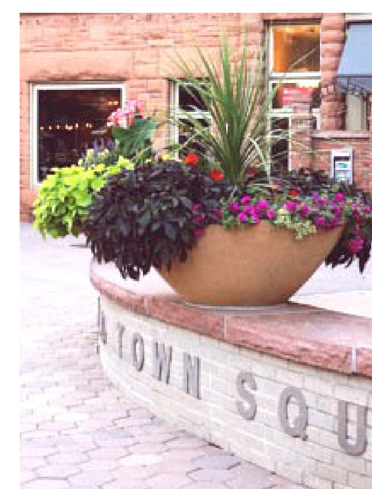
6 Blonde brick wall/stone cap w/ planter
