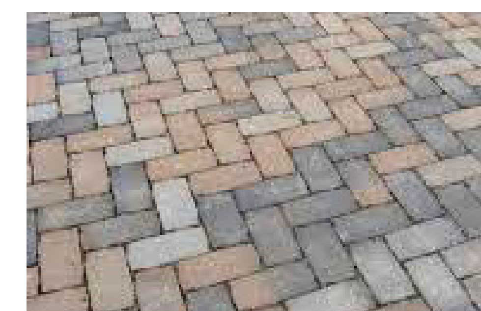
9 Concrete pavers - Herringbone pattern
