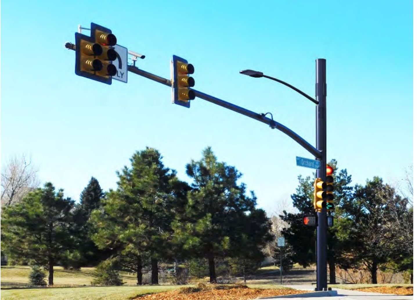
Figure 5: Example traffic signal mounted small cell
