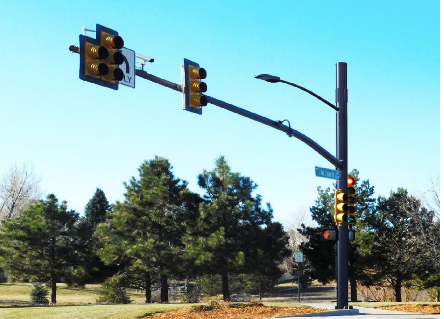
Figure 15: Example traffic signal mounted small cell
