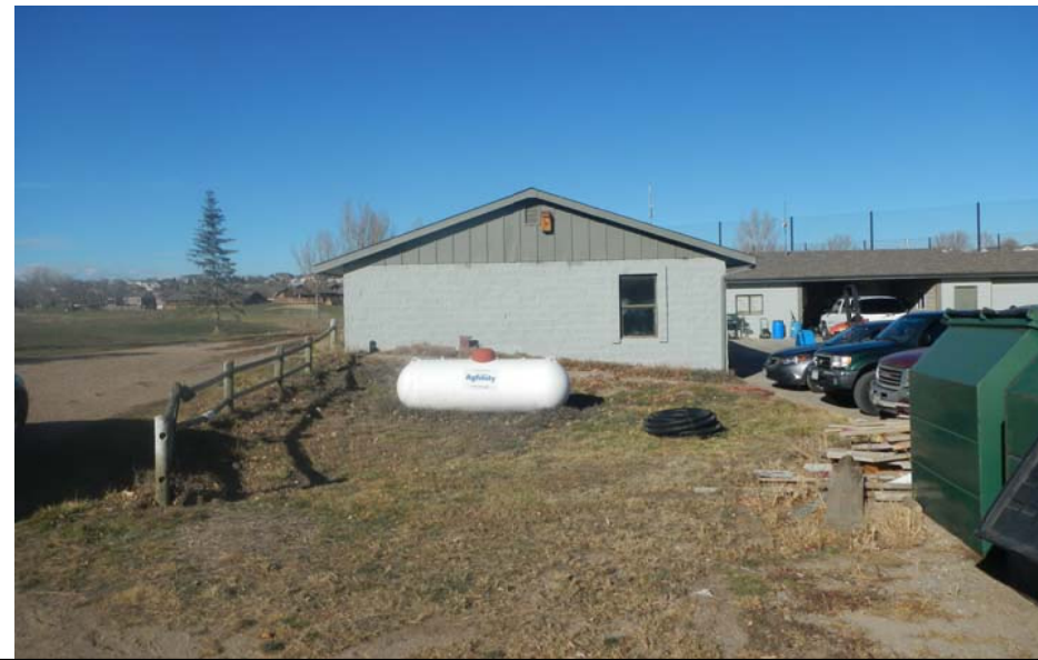
3 EXISTING SITE CONDITIONS AT NEW VZW SITE
