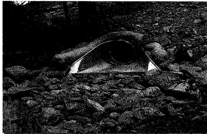
Photograph TOP-1. Riprap outlet protection.
