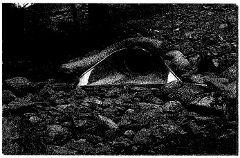
Photograph TOP-1. Riprap outlet protection.
