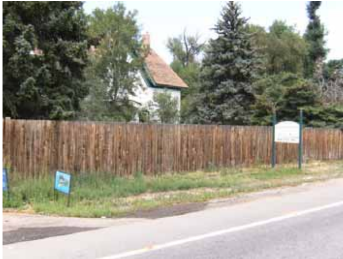
Looking at the Inverness Stock Farm house from the intersection of Vine Drive and Jerome
