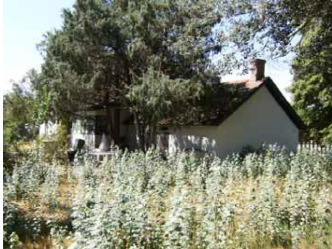
Inverness Stock Farm house north elevation – rear
