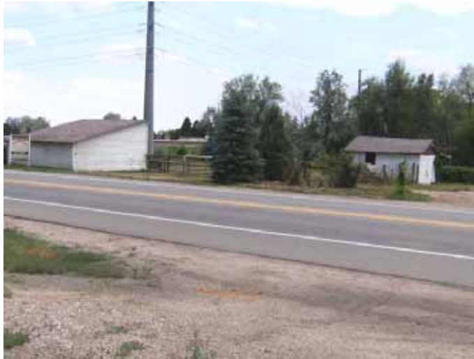
Existing outbuildings on the south parcel – these are east of the house shown above.
