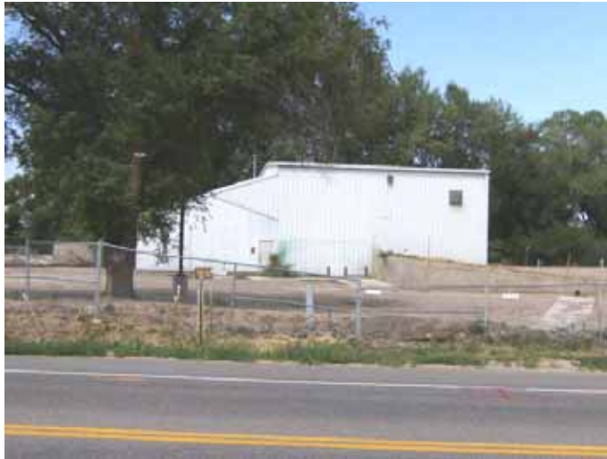
View from the most eastern point of south parcel looking due north
