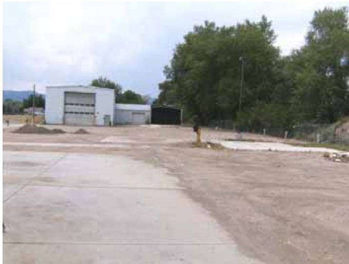
Looking west at the outbuilding west of the old Waste Management building
