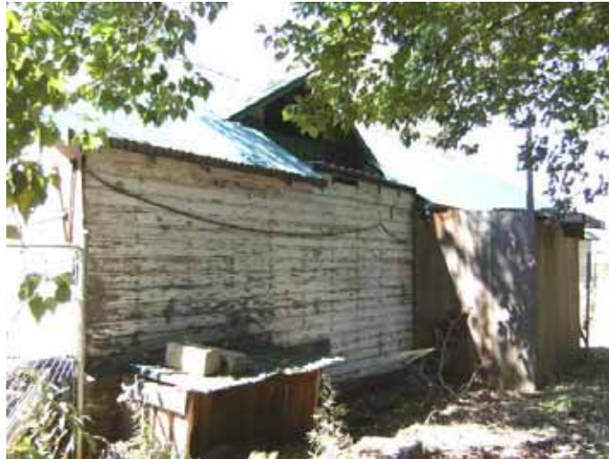
Rear of outbuilding on Inverness Stock Farm property
