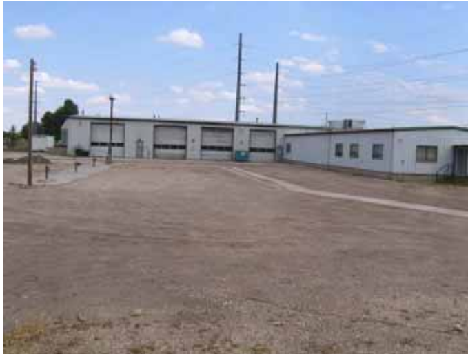
Looking east at the old Waste Management building
