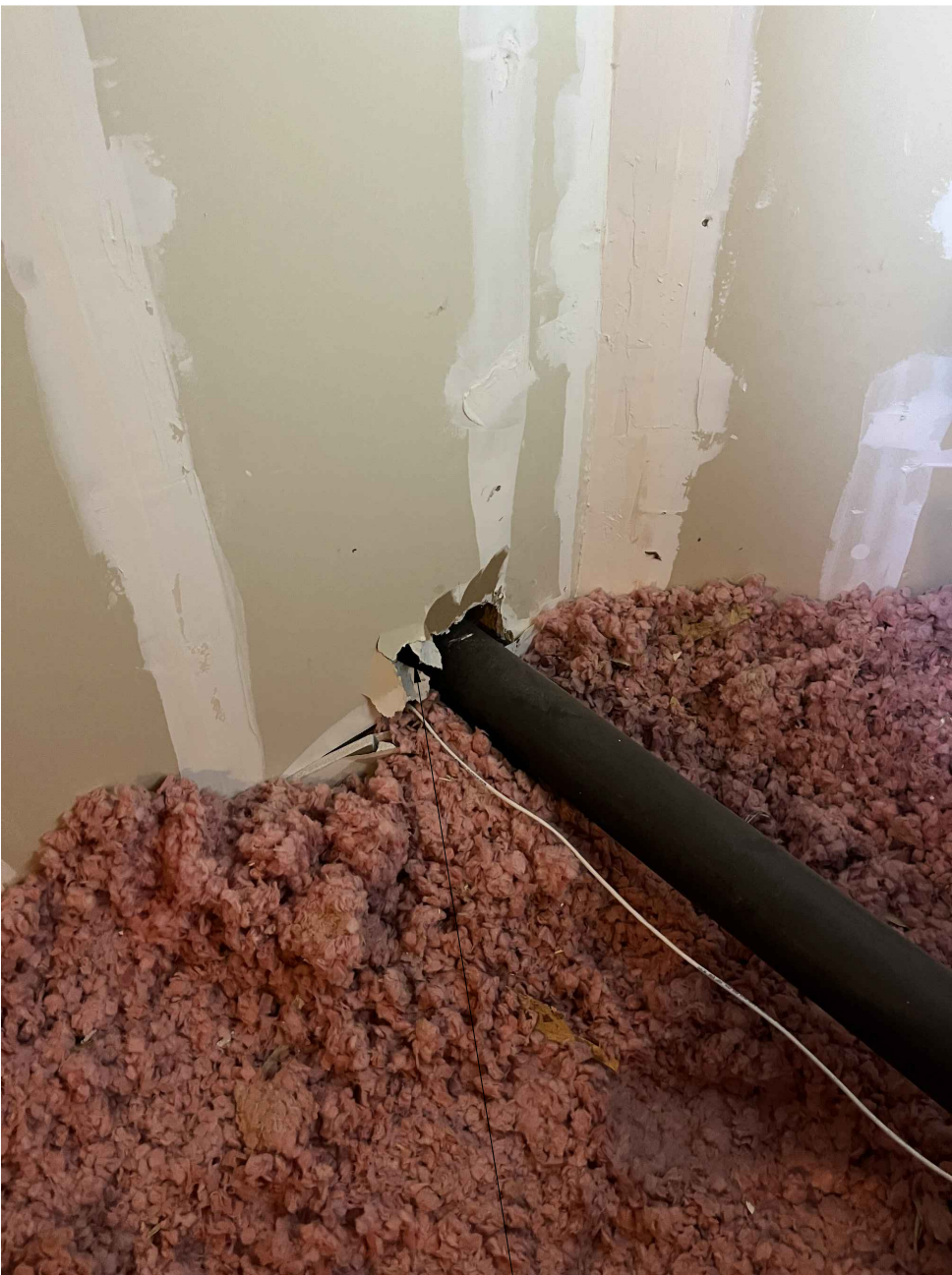
REPAIR DRYWALL AND INSTALL 3M FIRE CAULK
