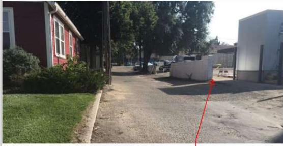
Historic stormwater sheet flow outlet
