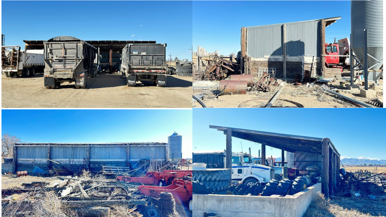
Building ID 505 Farm utility loading shed, pole building, built in 1970, low quality, 1.044 sf Age: 54 years
