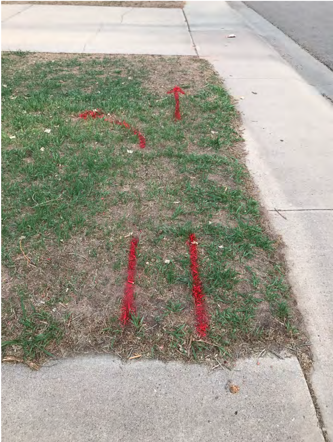
Utility Locate Photo #7
