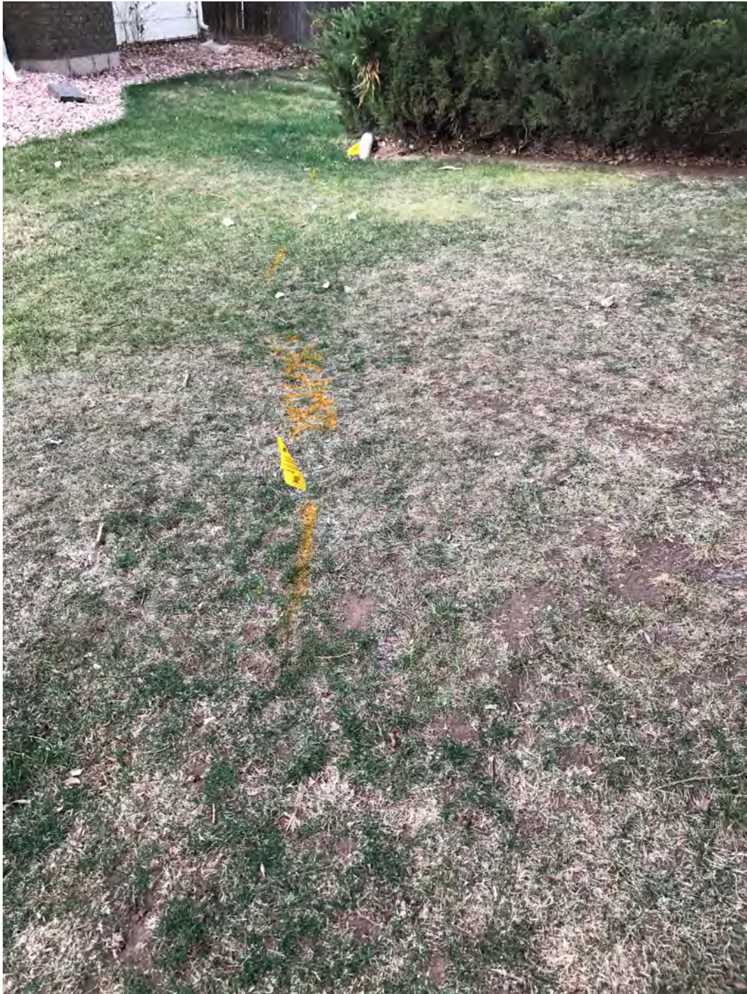
Utility Locate Photo #5
