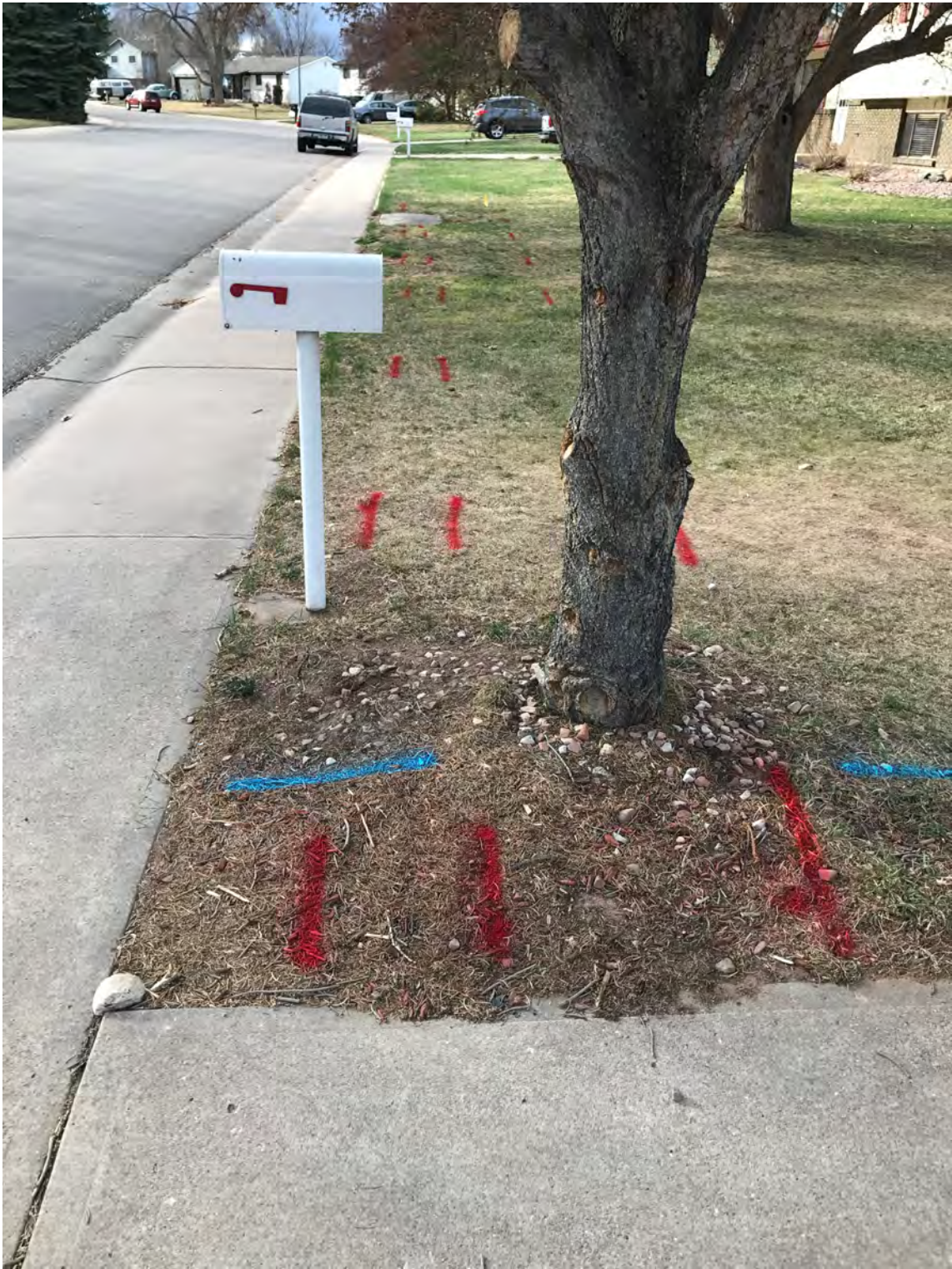
Utility Locate Photo #2
