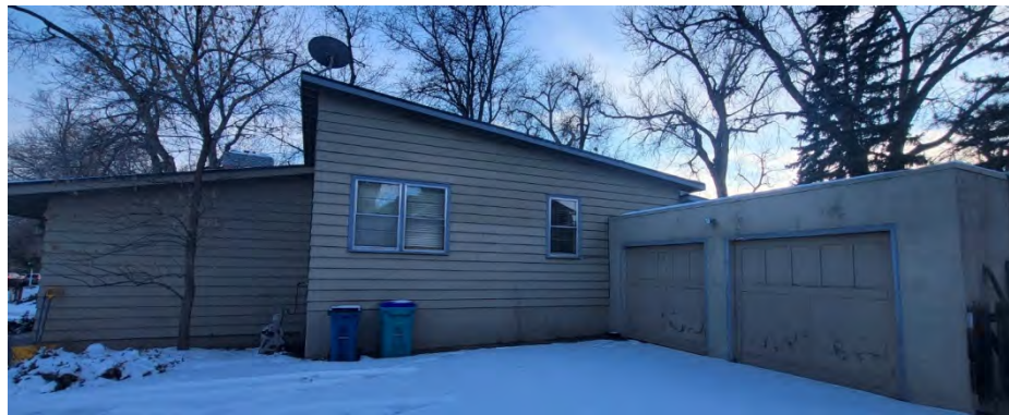
2. North Elevation House East Garage
