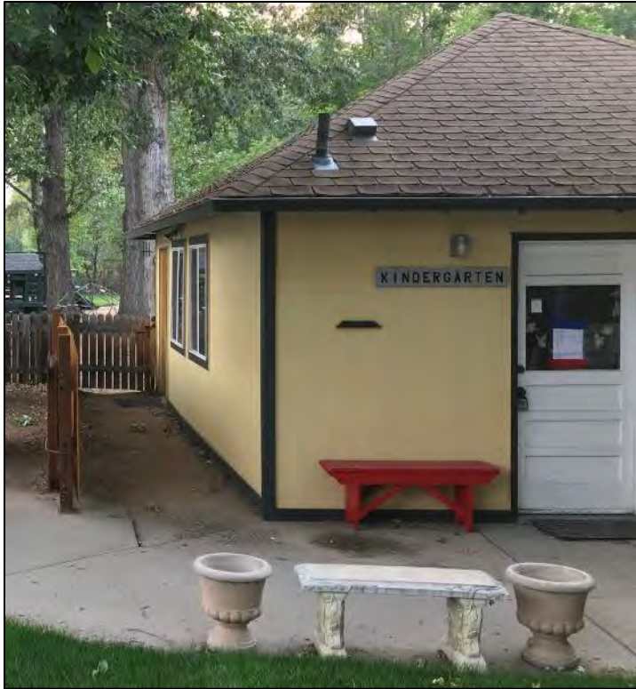
East Side Pre-Repair
