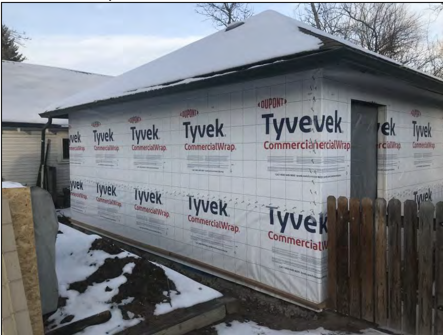
West Side Mid-Repair
