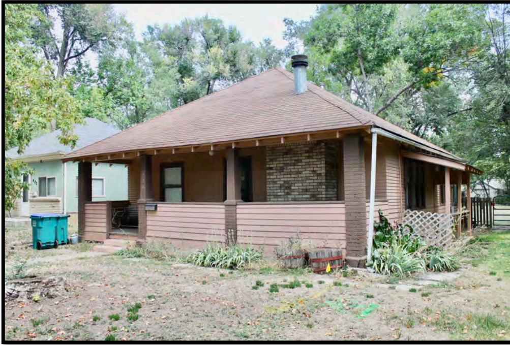
West Façade and South Wall, View to the Northeast
