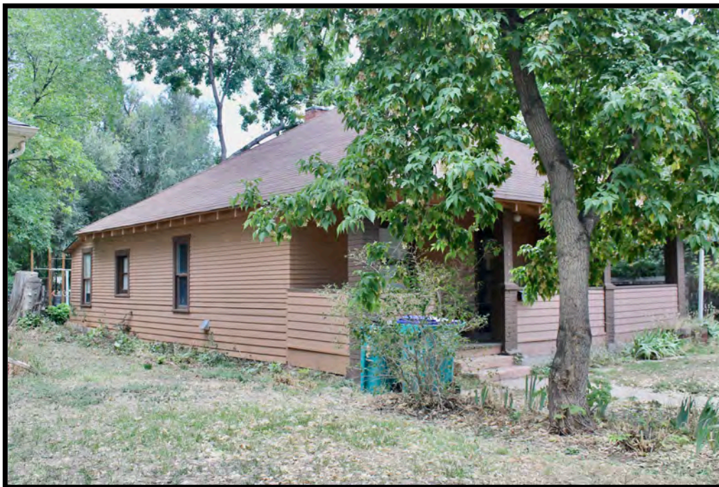
West Façade and North Wall, View to the Southeast
