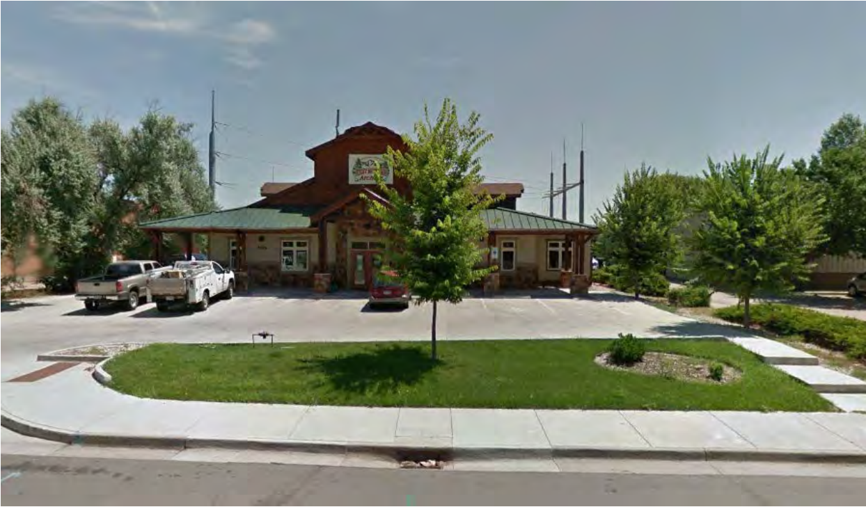
NORTH VIEW OF PROPERTY FOR PROPOSED TOWER LOCATION
