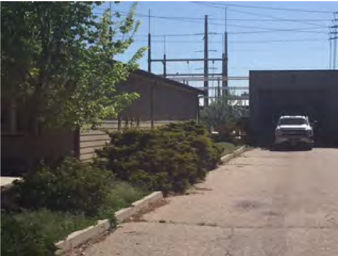
NORTH SIDE OF PROPERTY LOOKING WEST
