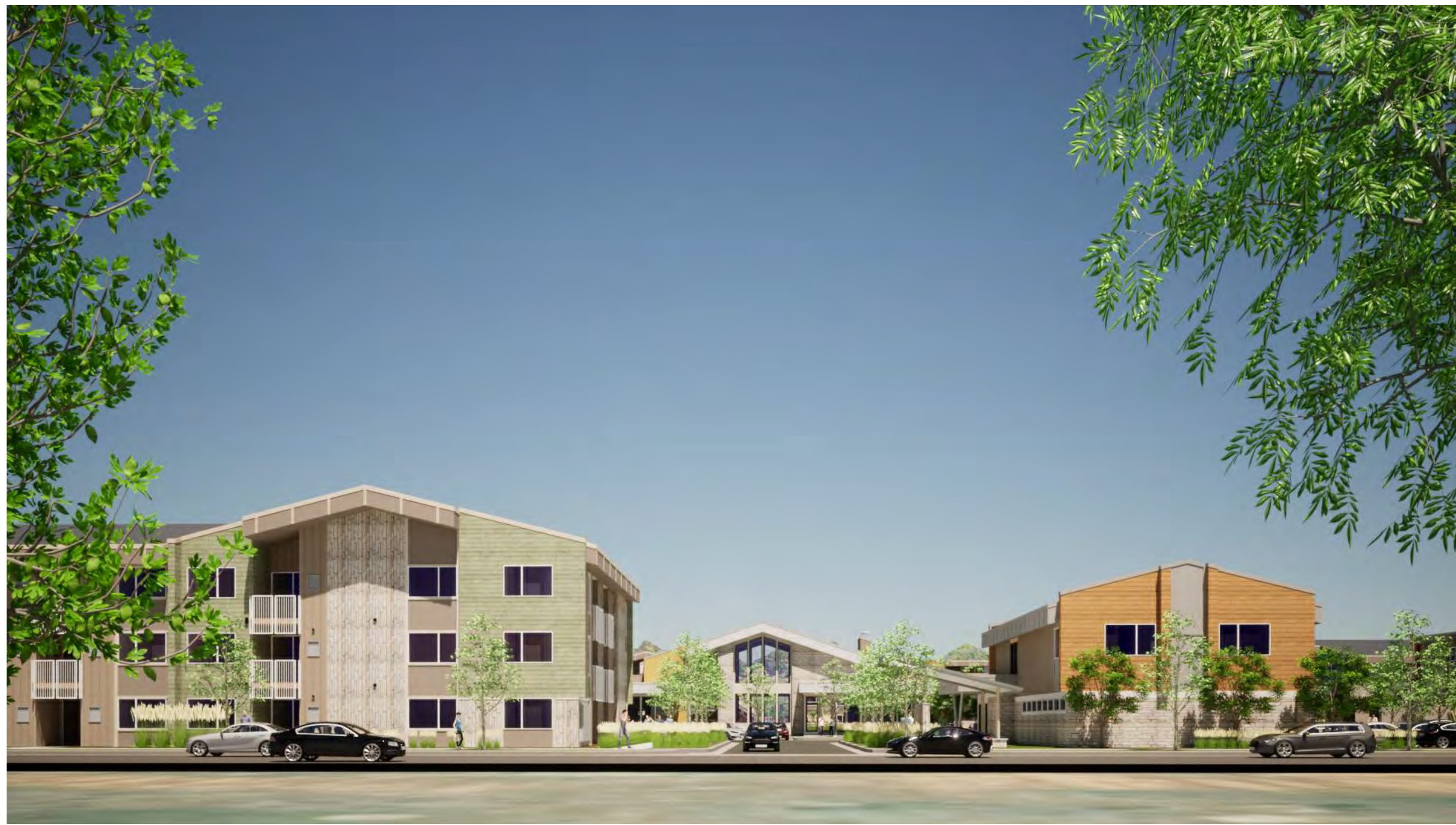
MAIN ENTRY - LOOKING SOUTH
