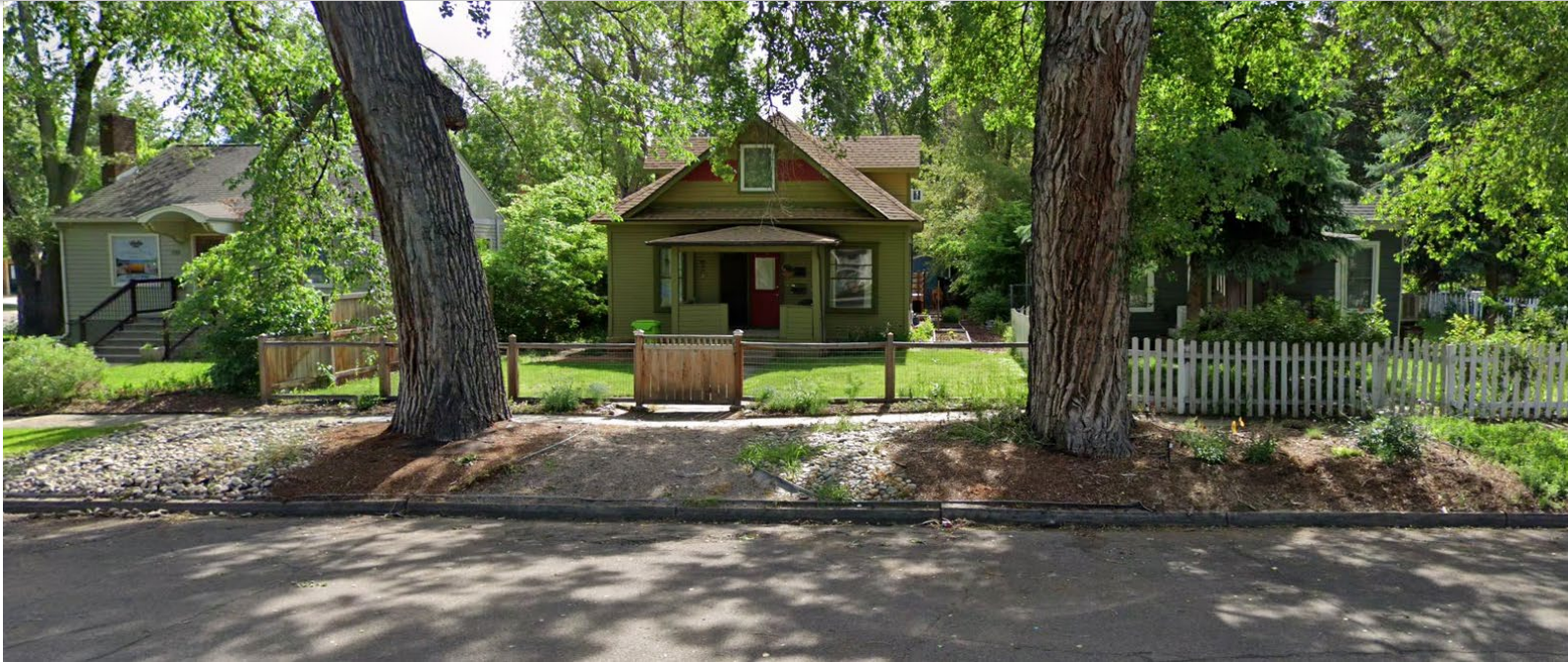
Front View from Whitcomb Street of Existing Two-Family Home
