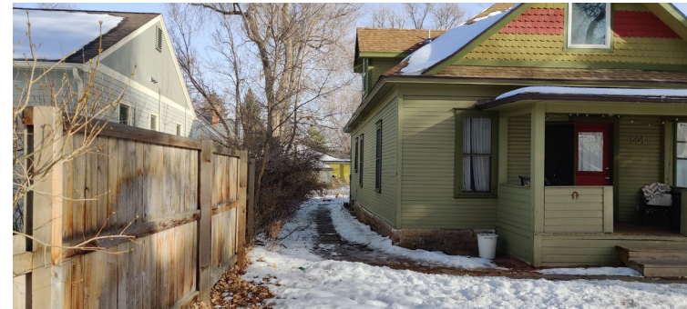
Front view of connecting walk
