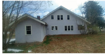
EXISTING CONDITIONS - WEST
