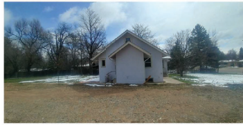
EXISTING CONDITIONS - WEST
