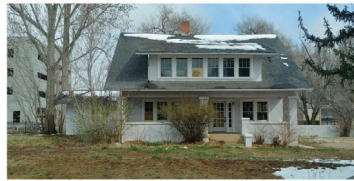
EXISTING CONDITIONS - SOUTH
