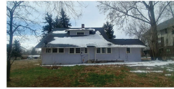
EXISTING CONDITIONS - NORTH
