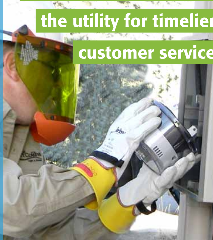
>> Installation of new Advanced Meters
