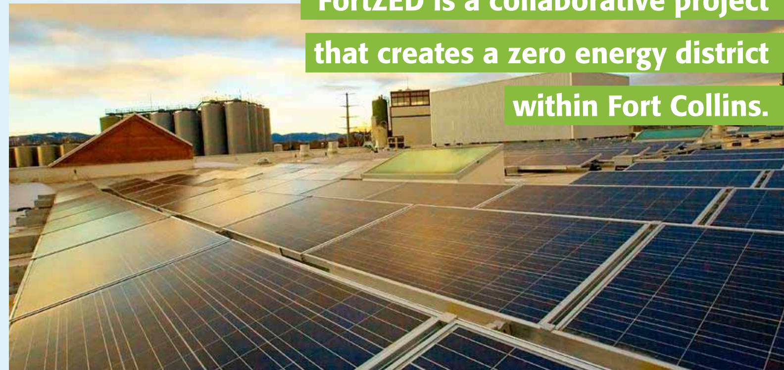
>> Solar PV on New Belgium Brewing
