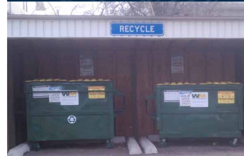
>> New recycling enclosure at Heatheridge Lakes Condos
