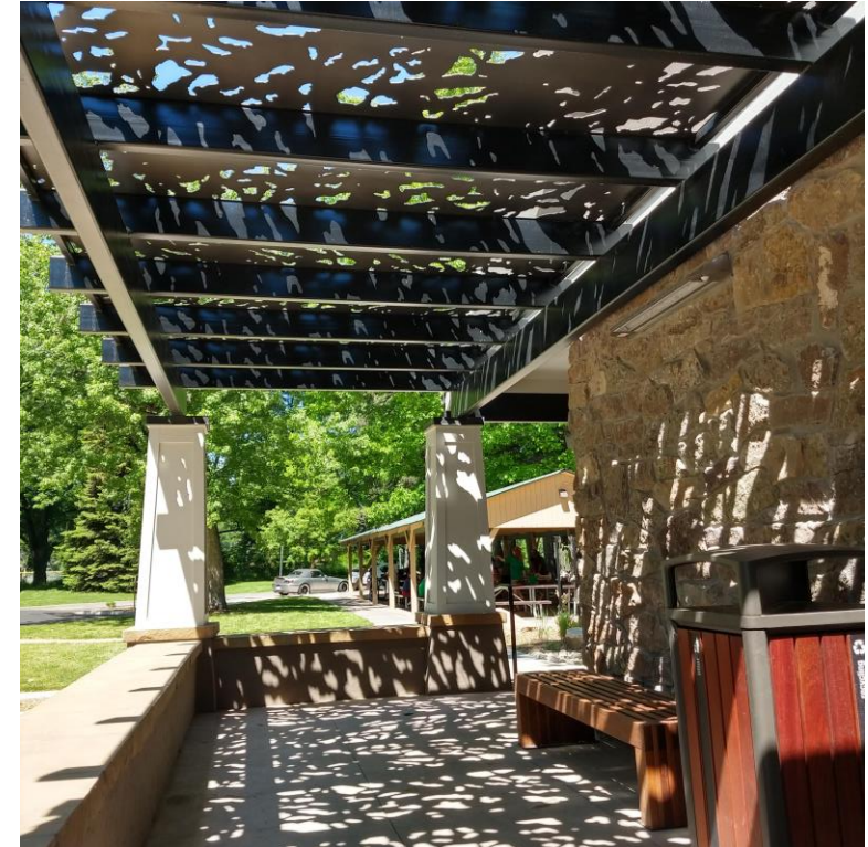
City Park Restroom
