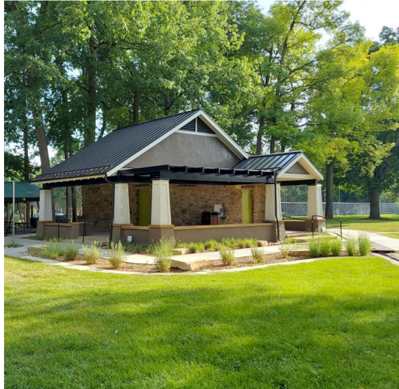
City Park Restroom
