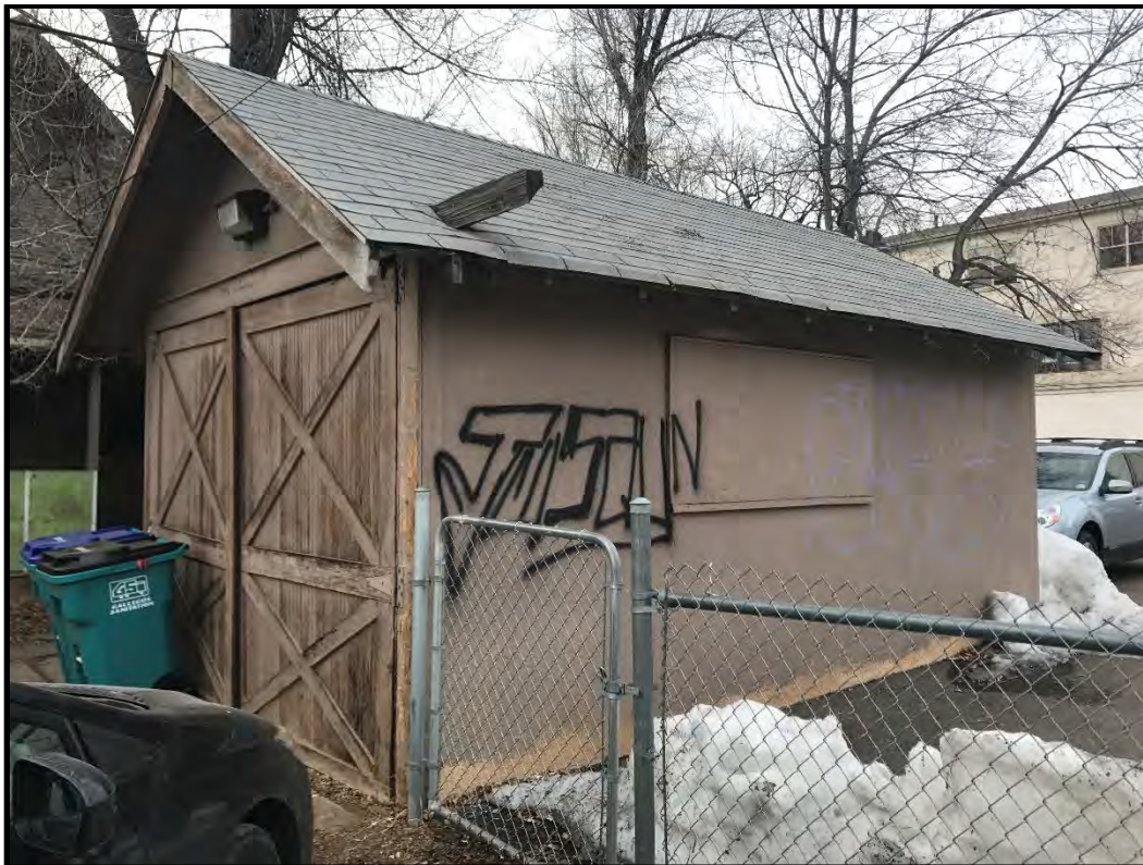
724 South College Avenue, detached garage, looking northwest.
