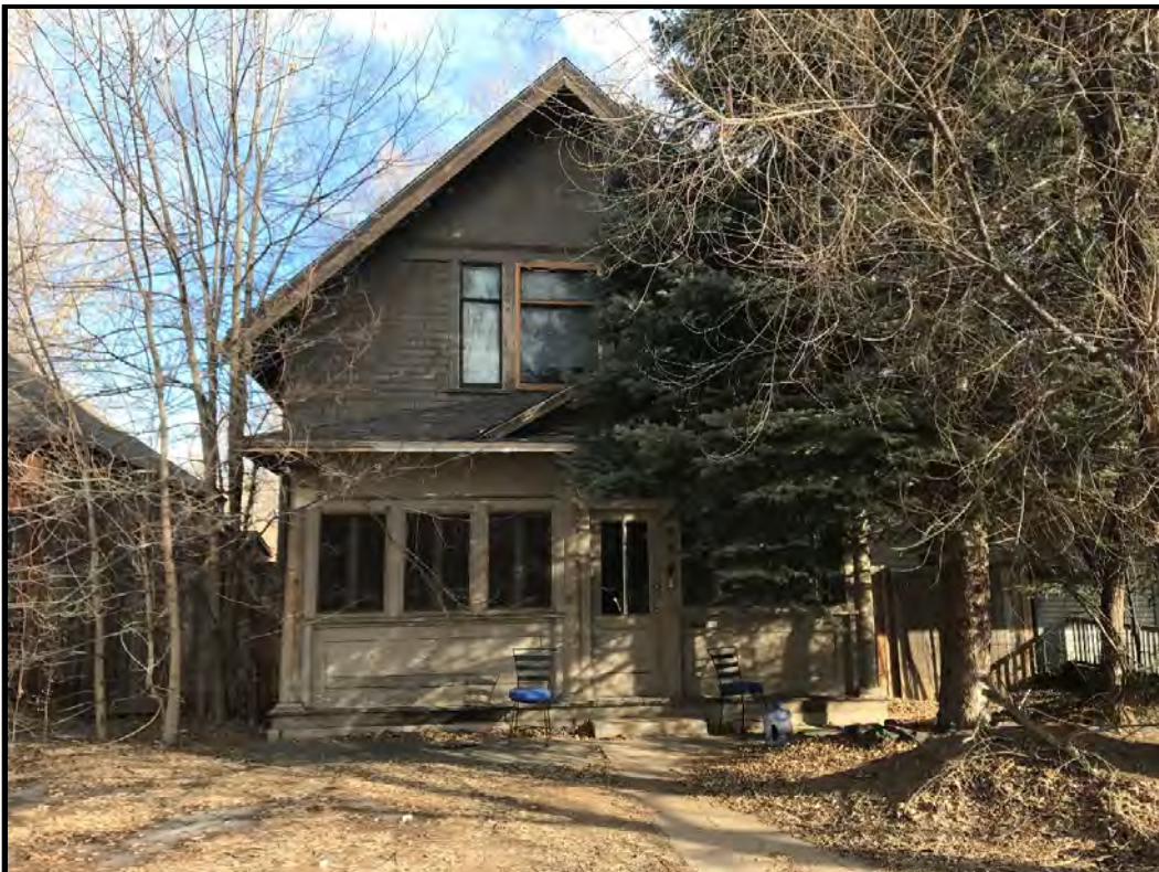
724 South College Avenue, façade, looking east.
