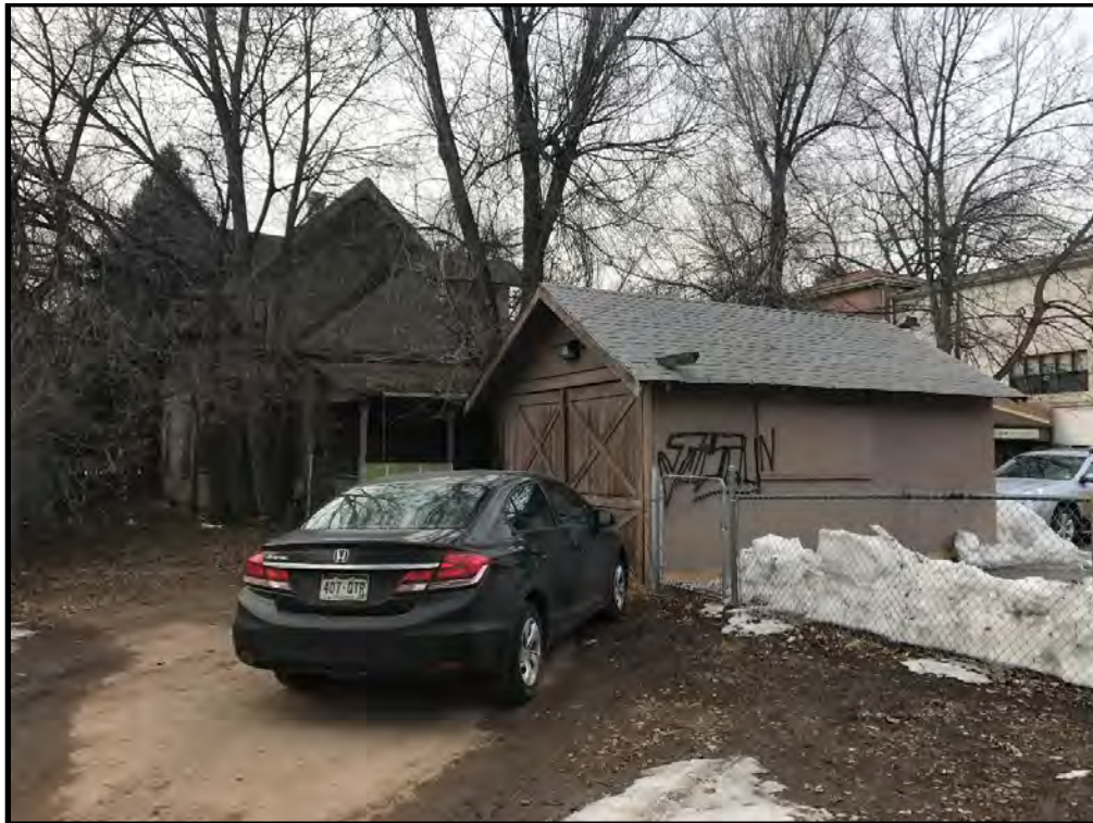
724 South College Avenue, detached garage behind house, looking northwest.
