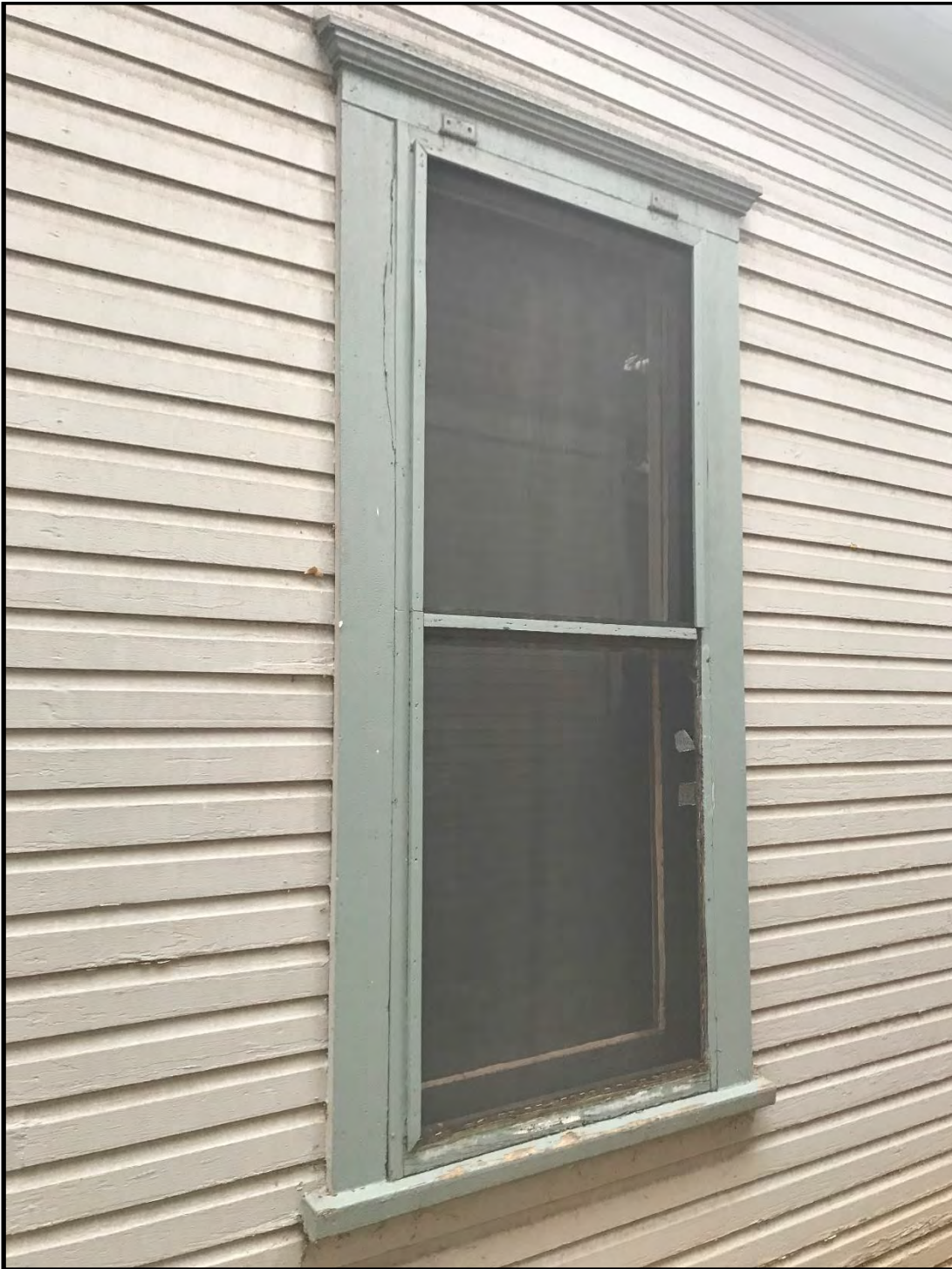
726 South College Avenue, smaller double-hung window on north elevation, looking southwest.
