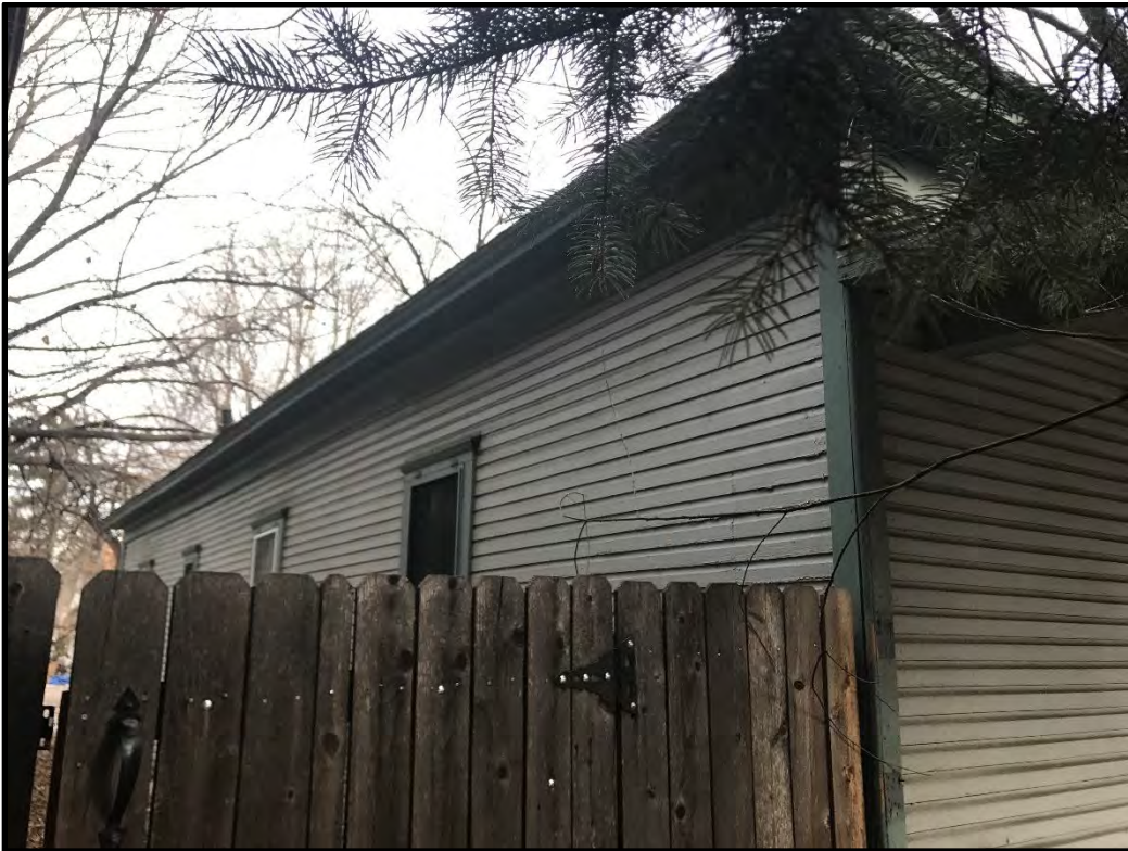
726 South College Avenue, north elevation, looking southeast.
