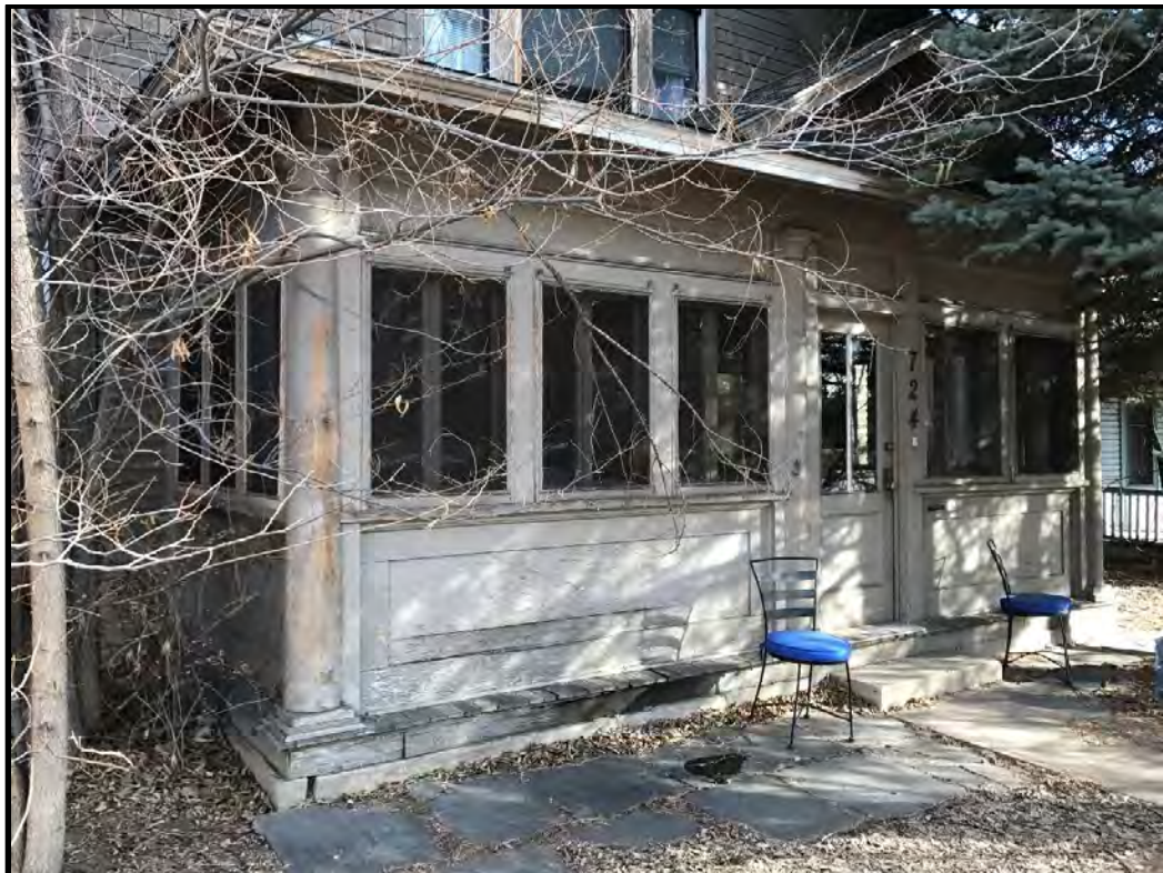
724 South College Avenue, enclosed front porch, looking southeast.
