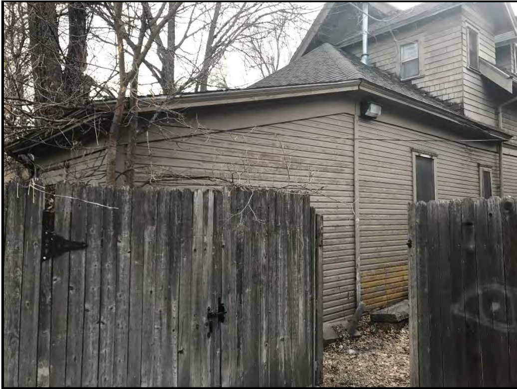
724 South College Avenue, closer view of rear wing, looking southwest.
