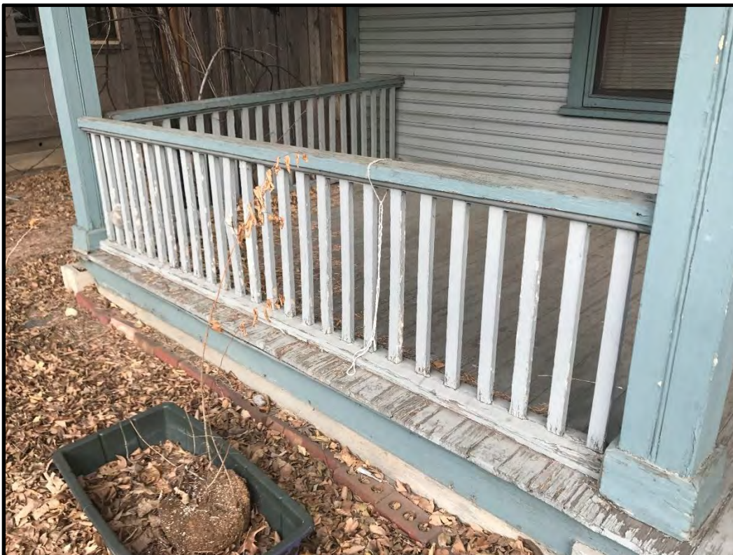
726 South College Avenue, balustrade front porch railing, looking northeast.
