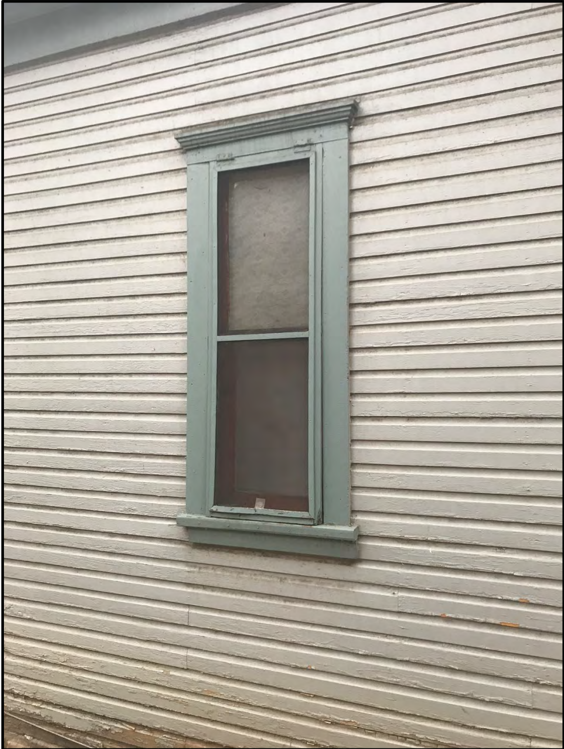
726 South College Avenue, small double-hung window on north elevation, looking southeast.
