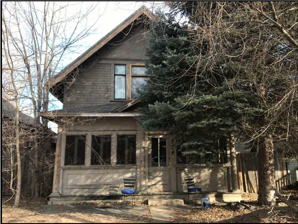
724 South College Avenue, façade, looking east.
