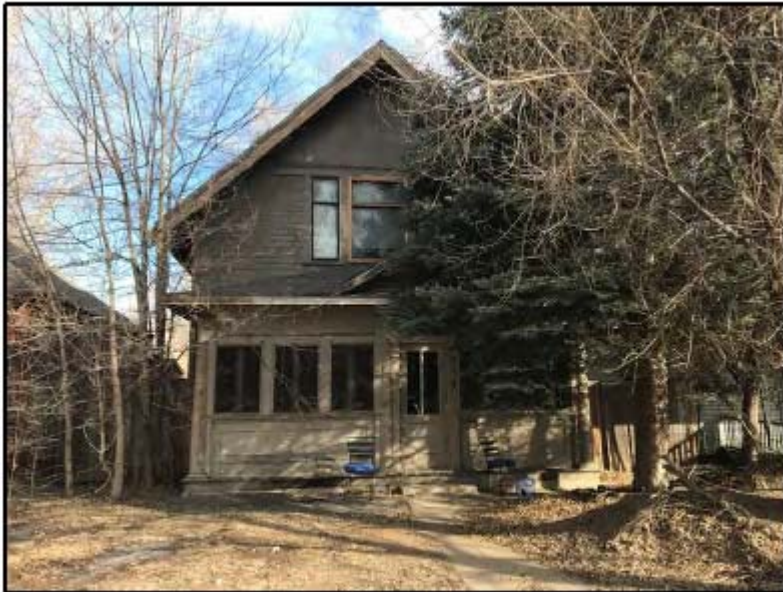
724 South College Avenue, façade, looking east.
