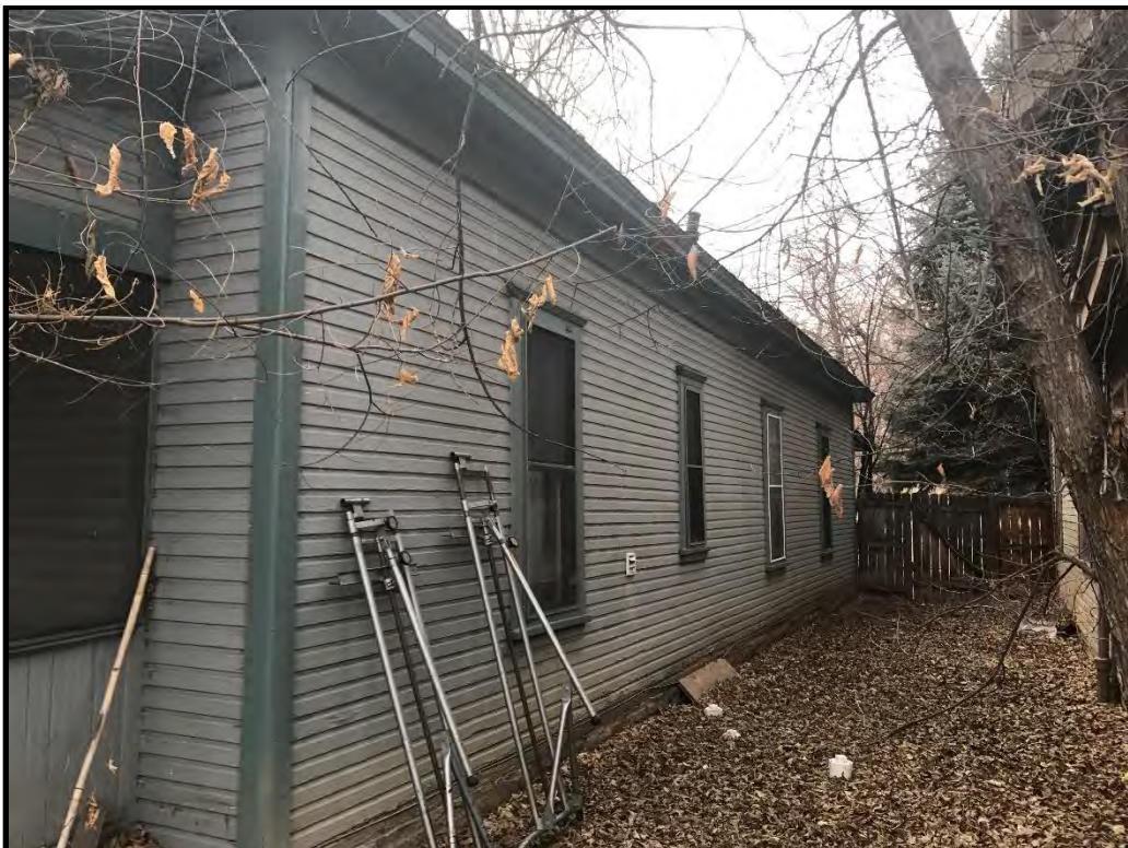
726 South College Avenue, south elevation, looking east-northeast.
