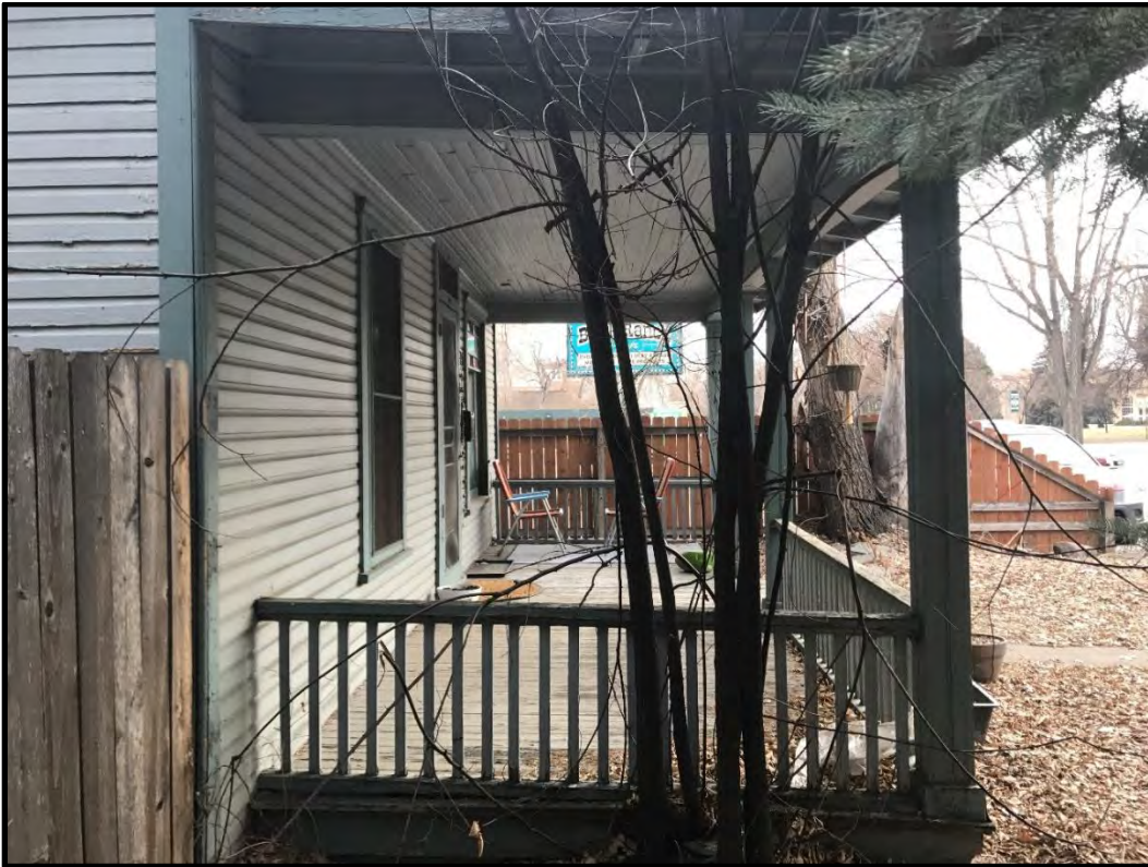
726 South College Avenue, open front porch, looking south.
