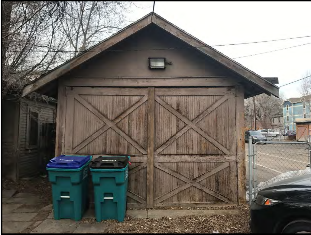
724 South College Avenue, front/south side of detached garage, looking north.
