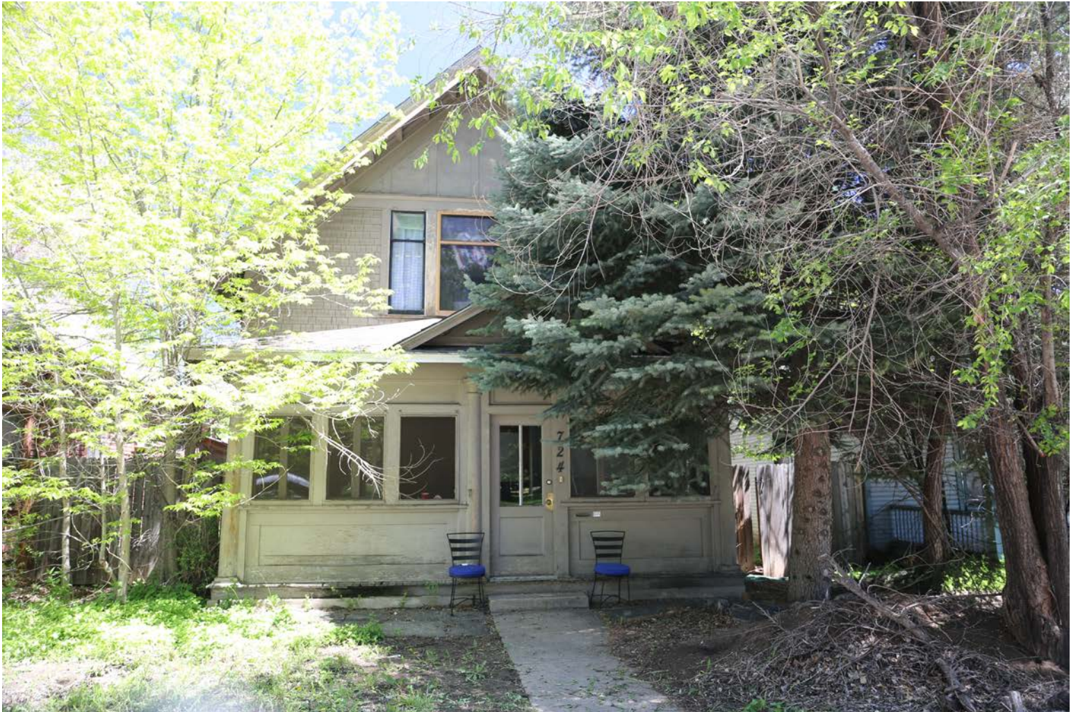
View of west (front) wall looking east
