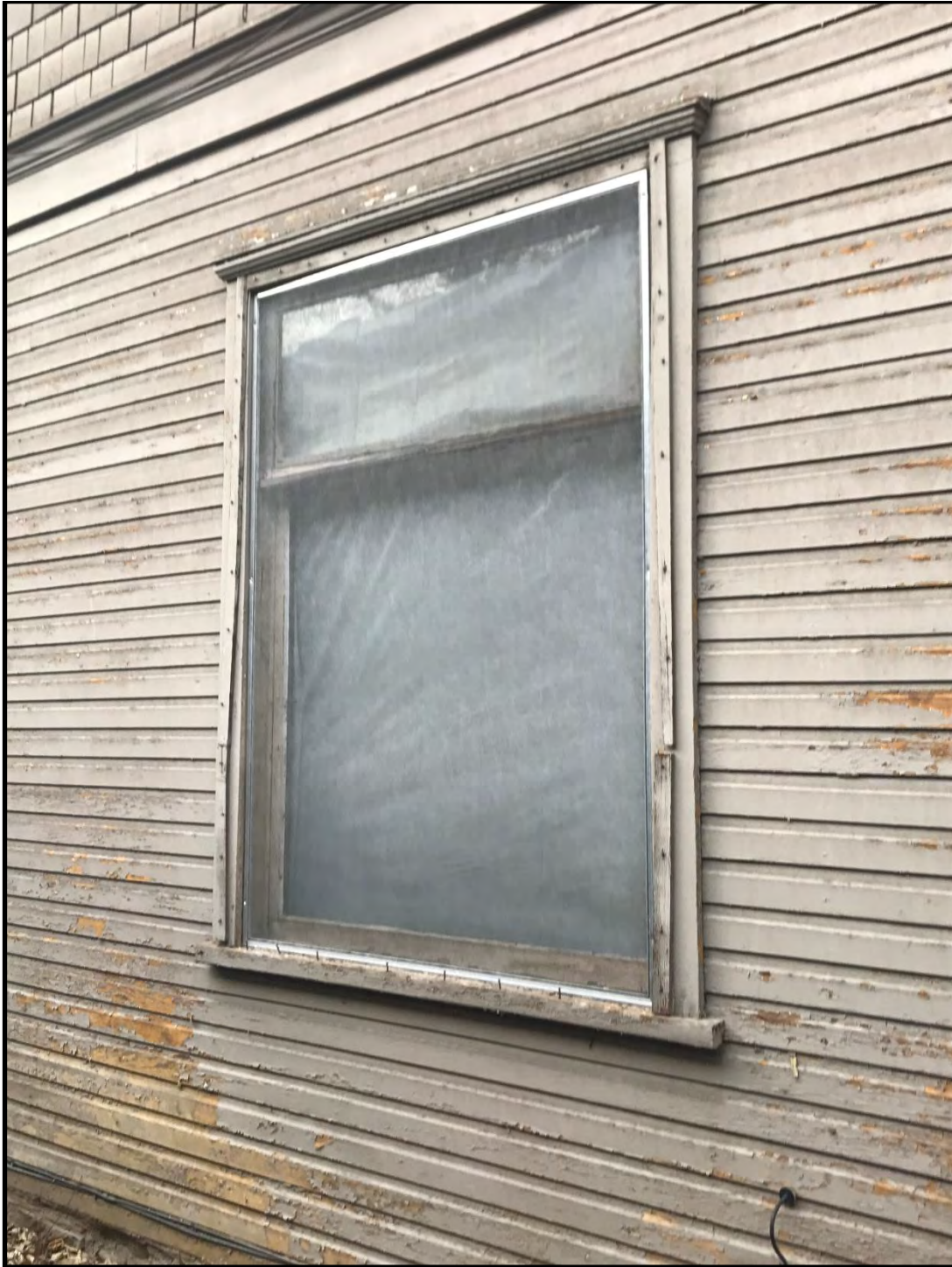
724 South College Avenue, large sash-and-transom window on south elevation.
