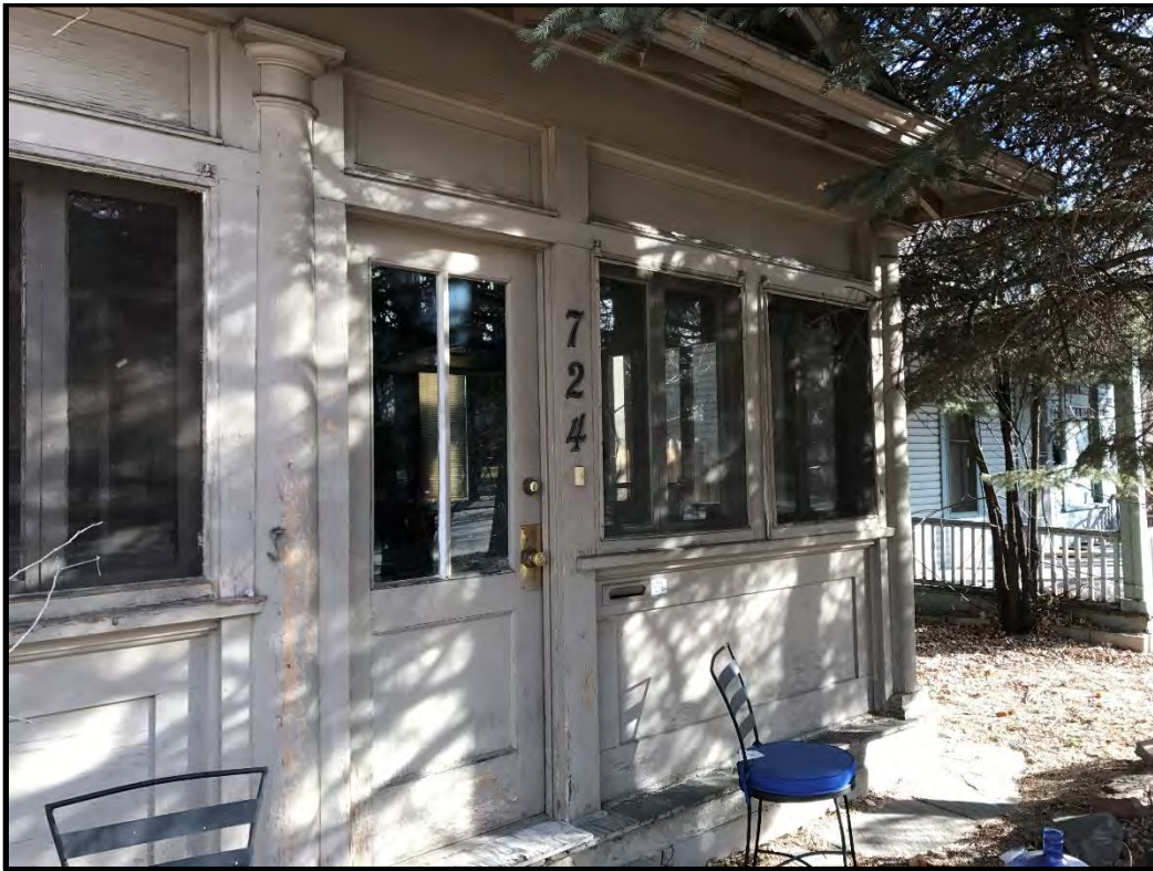
724 South College Avenue, right side of enclosed front porch, looking southeast.
