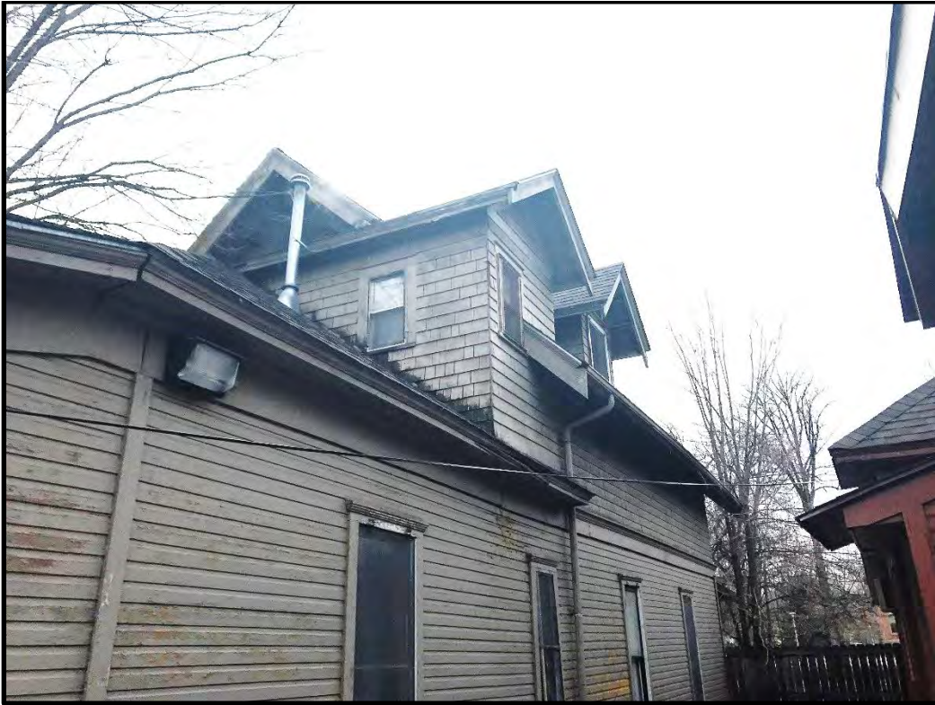
724 South College Avenue, east elevation dormers, looking southwest.
