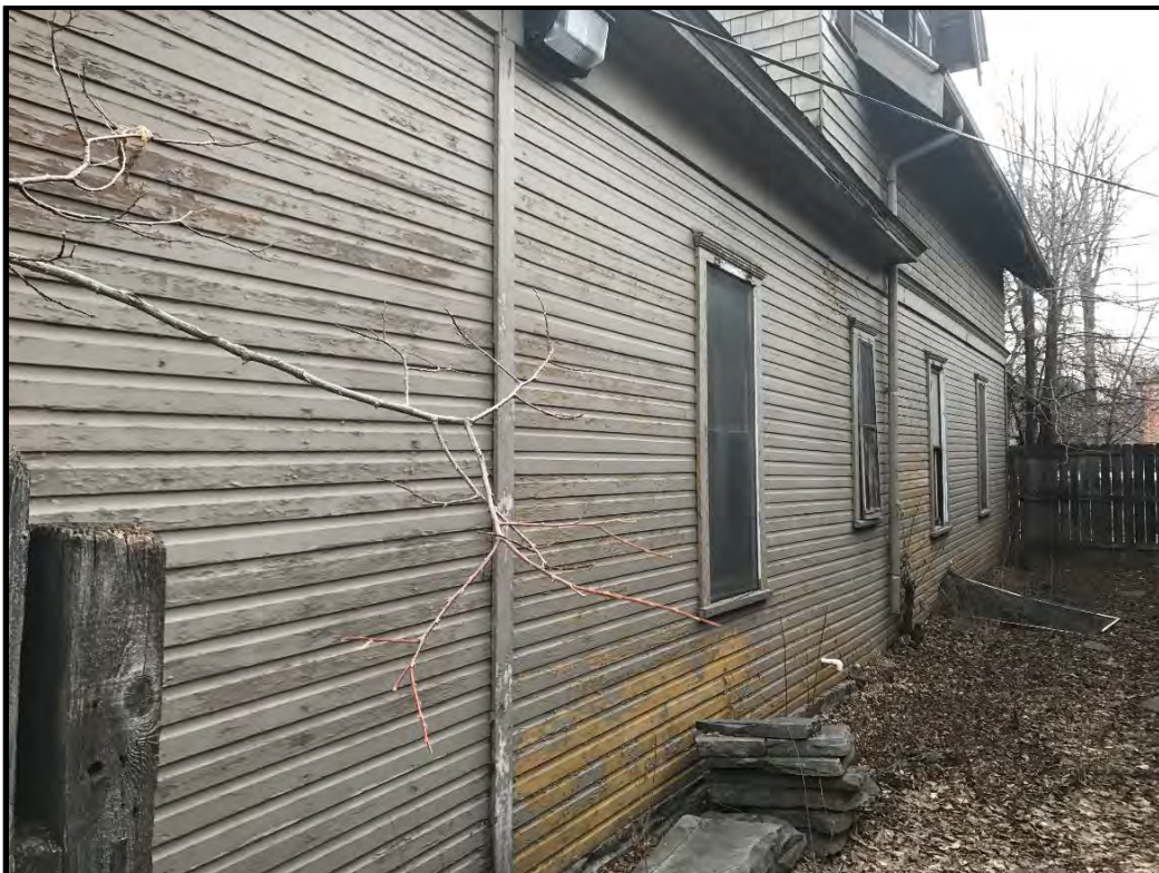
724 South College Avenue, north elevation, looking west-southwest.
