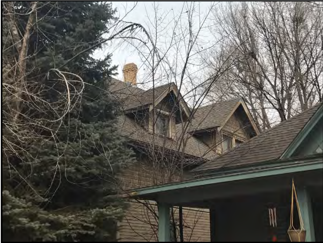
724 South College Avenue, south elevation dormers and yellow brick chimney stack, looking northeast.
