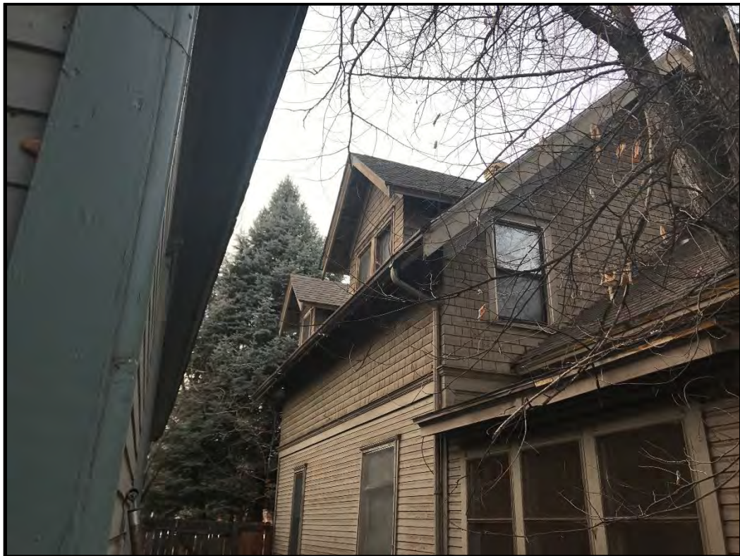
724 South College Avenue, south elevation, looking northwest.
