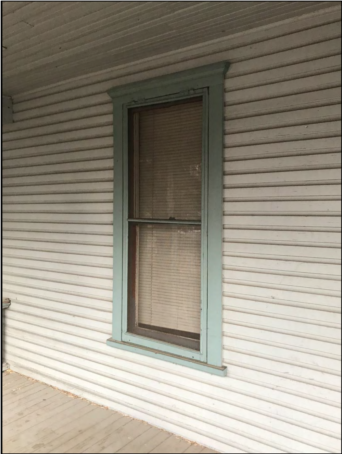
726 South College Avenue, double-hung window on facade, looking northeast.
