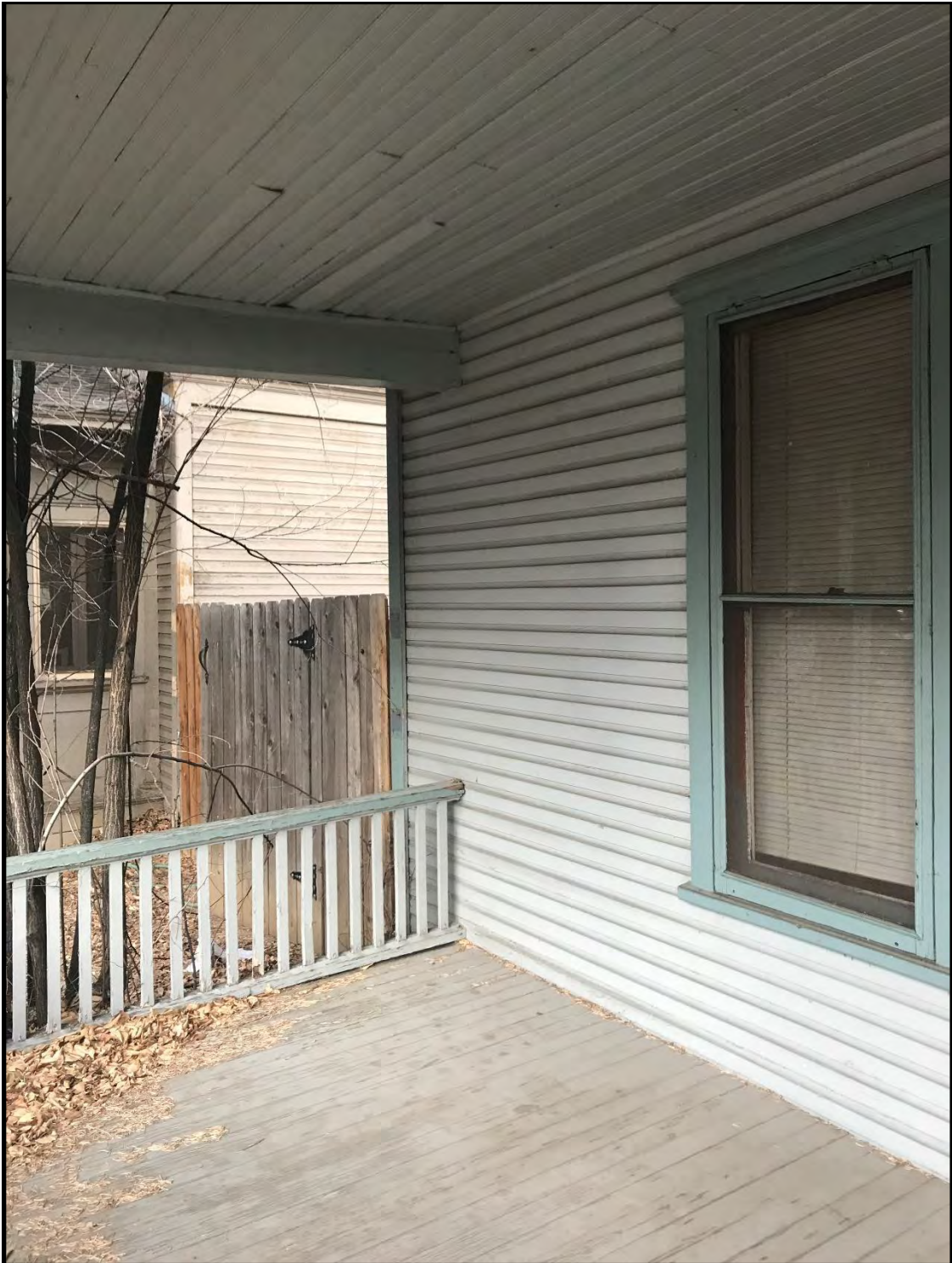
726 South College Avenue, north side of open front porch, looking northeast.
