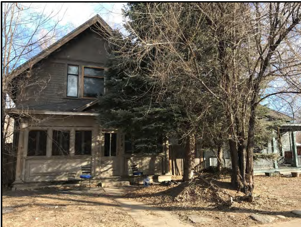
724 South College Avenue, looking ESE, with 726 South College Avenue visible to the right.
