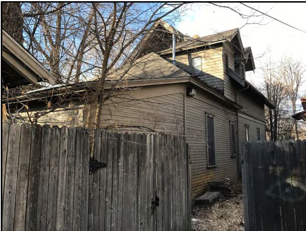
724 South College Avenue, north elevation and shed-roofed rear addition, looking west-southwest.
