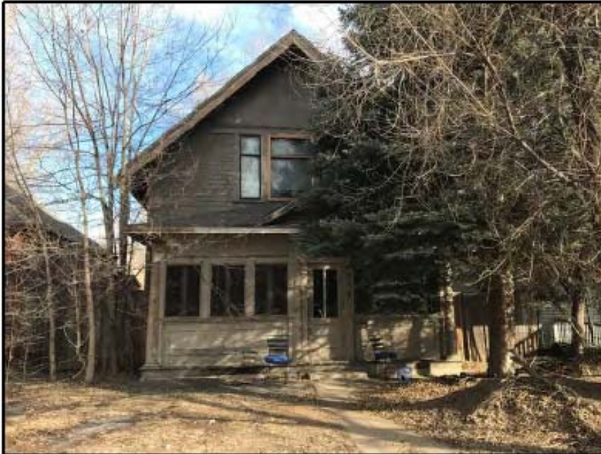
724 South College Avenue, façade, looking east.
