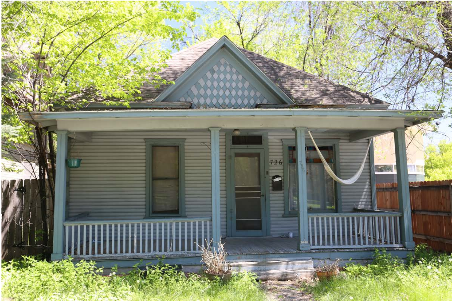
View of west (front) wall looking east
