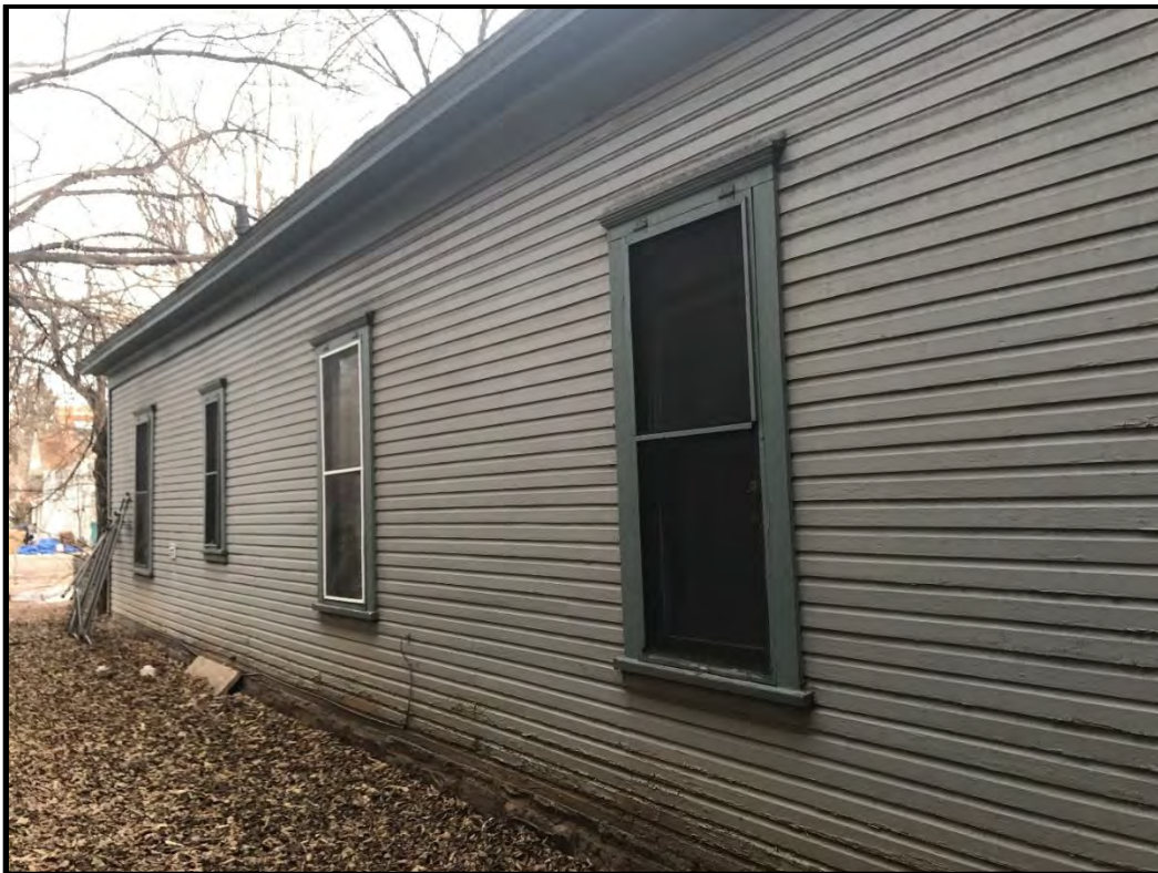
726 South College Avenue, north elevation, looking southeast.
