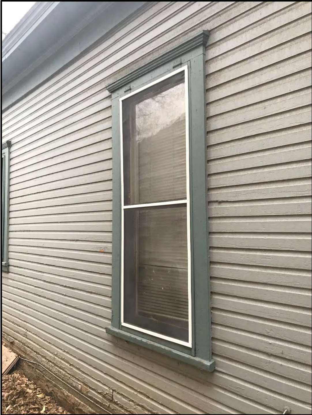
726 South College Avenue, large north elevation window, looking southeast
