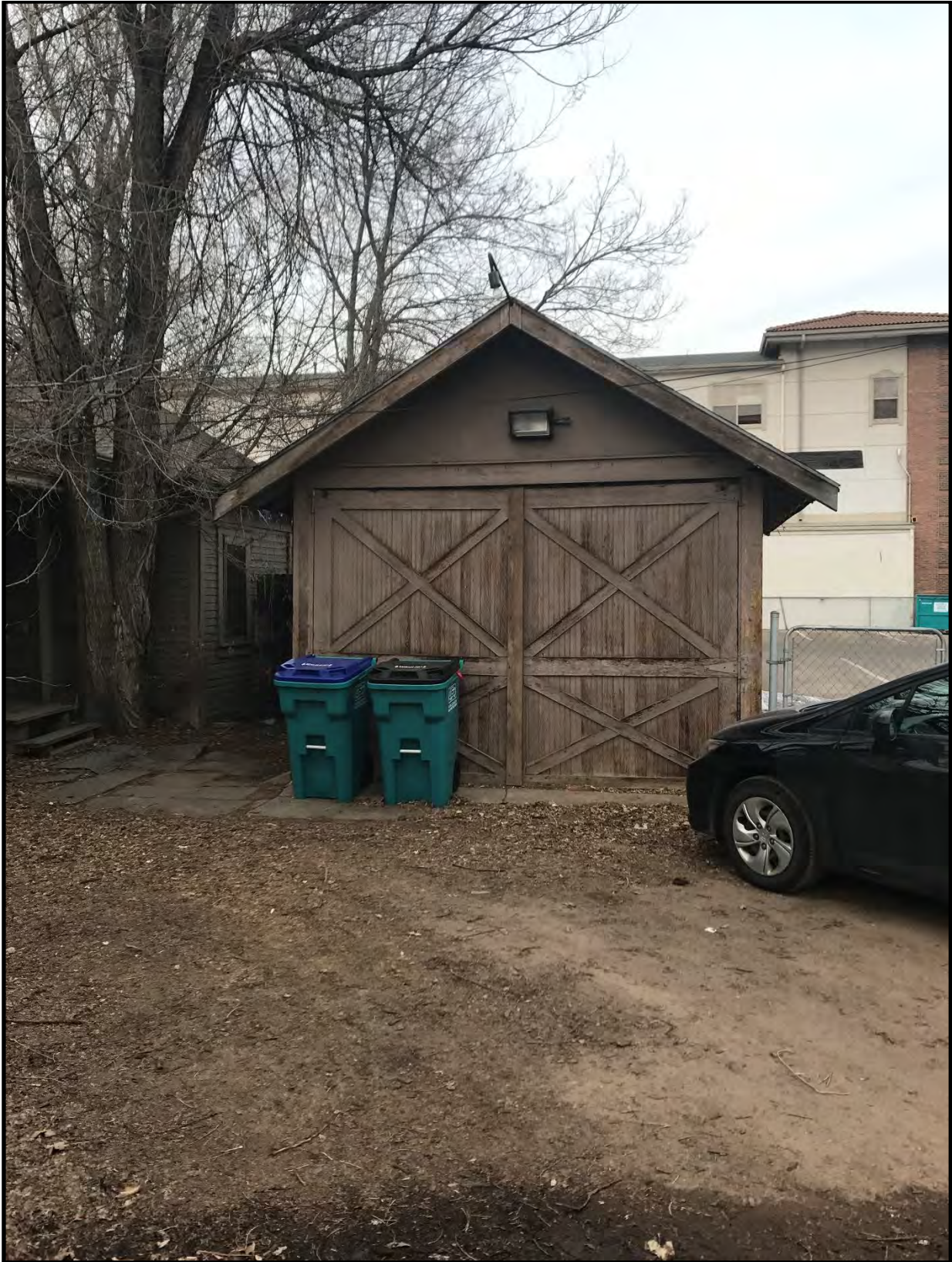
724 South College Avenue, detached garage, looking north.
