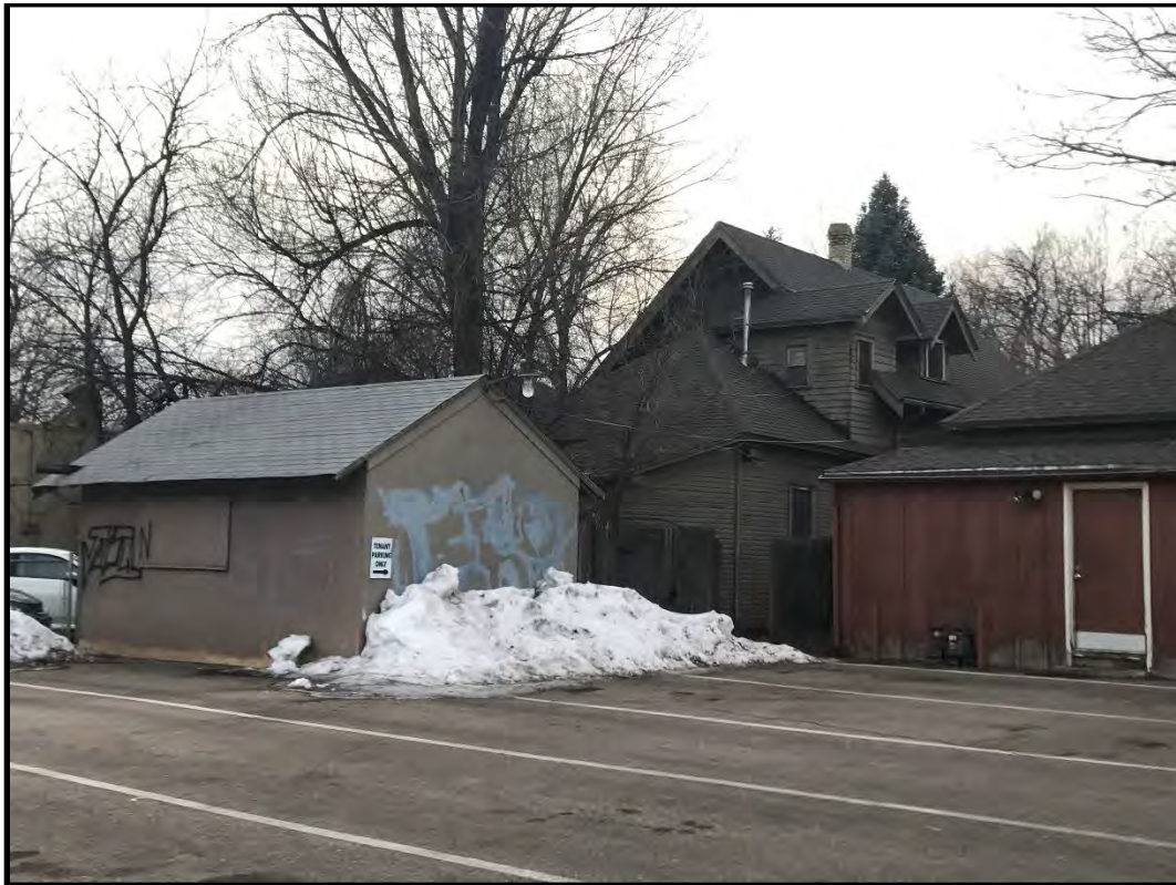
724 South College Avenue, detached garage behind house, looking southwest.
