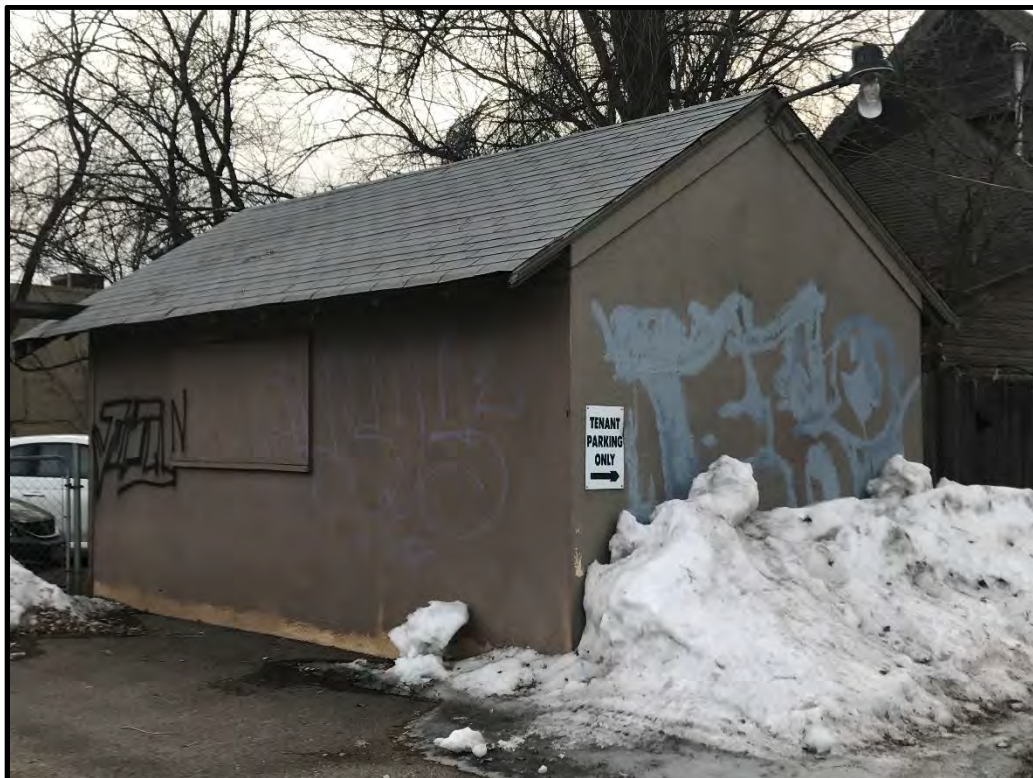
724 South College Avenue, detached garage, looking southwest and showing sealed window.
