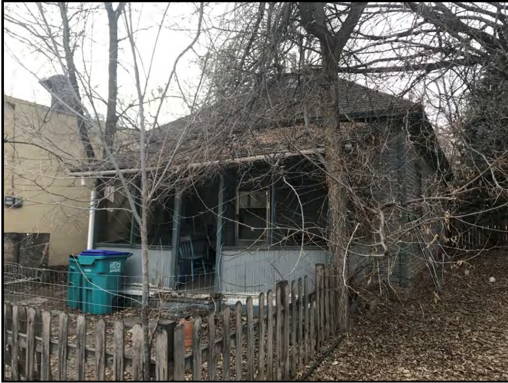
726 South College Avenue, rear elevation, looking southwest.
