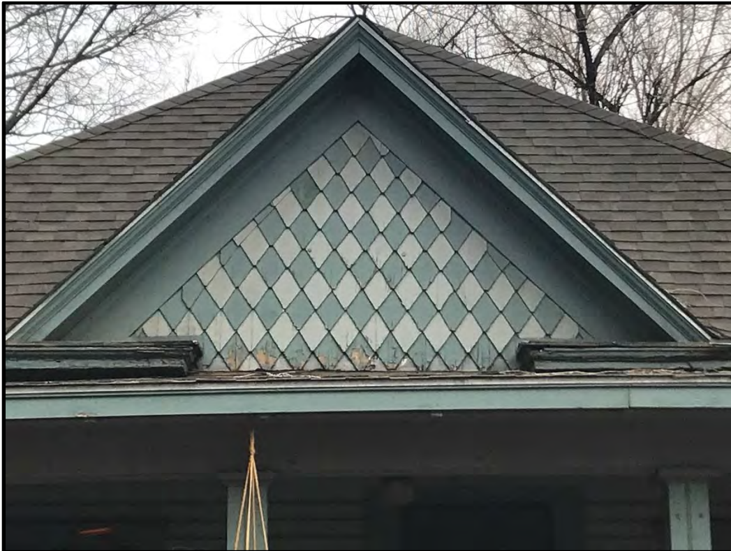
Small shingle-clad gable of façade of 726 South College Avenue, looking east.
