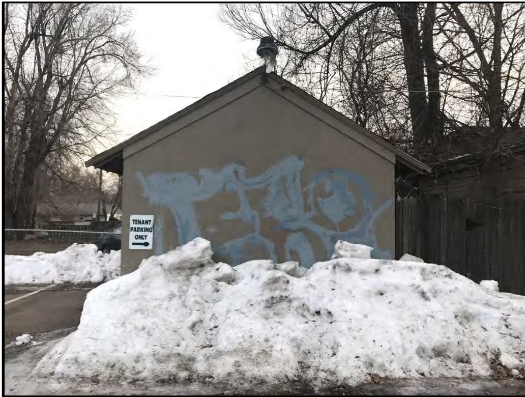
724 South College Avenue, north elevation of detached garage, looking south.
