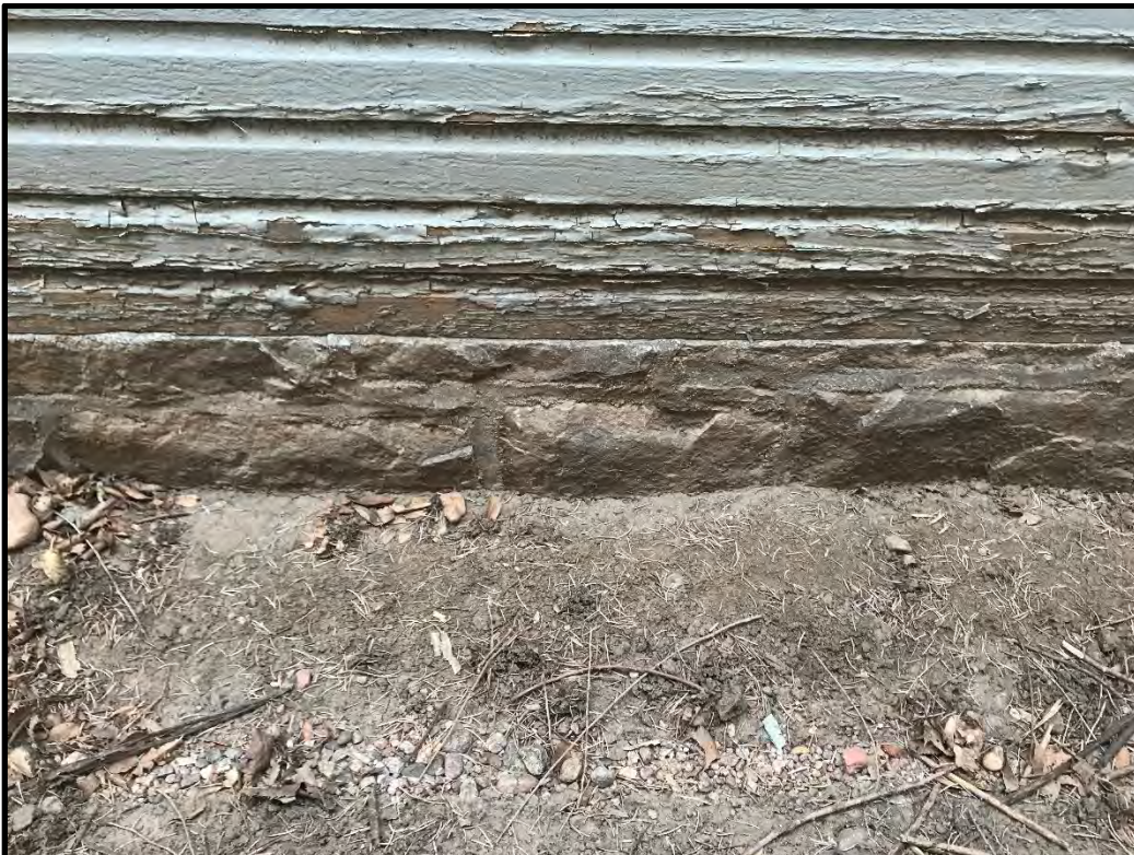
726 South College Avenue, exposed stone foundation.
