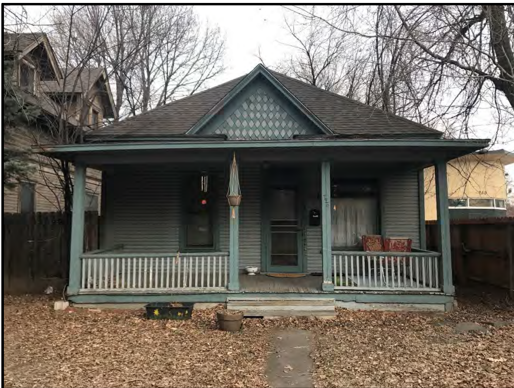
Closer view of 726 South College Avenue facade, looking east.
