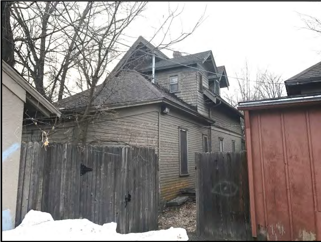
724 South College Avenue, rear/east and north elevations, looking southwest.
