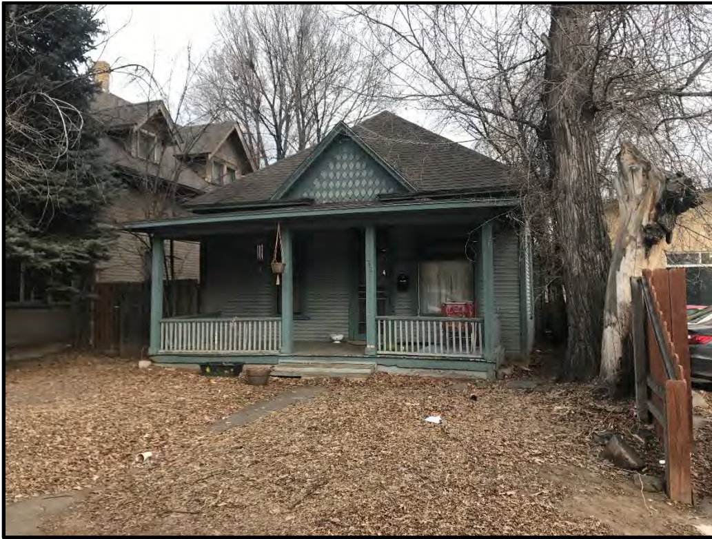
726 South College Avenue, looking east-northeast.
