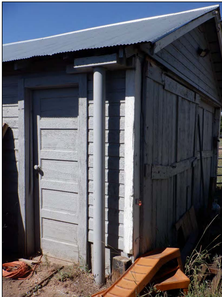
Figure 9: Feature 2, support post at northeast corner, view southwest (Image #629, RLS 8/23/2022).
