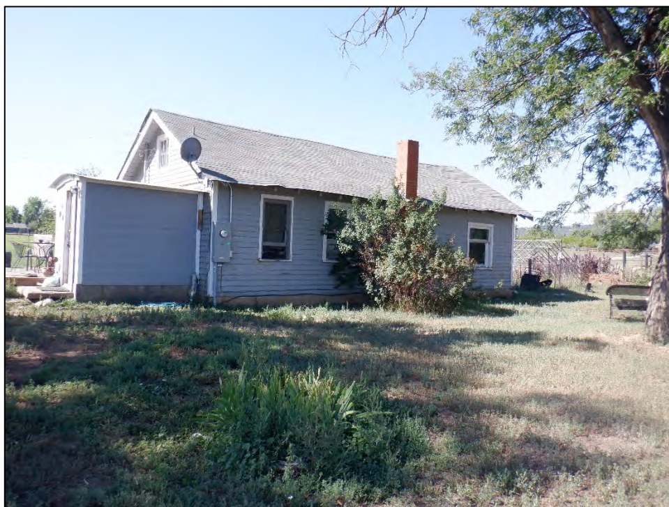
Figure 3: Feature 1, north elevation, view southwest (Image #612, RLS 8/23/2022).
