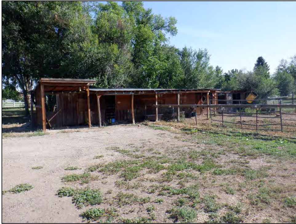
Figure 9: Feature 2, south elevation, view northeast (Image #597, RLS 8/23/2022).
