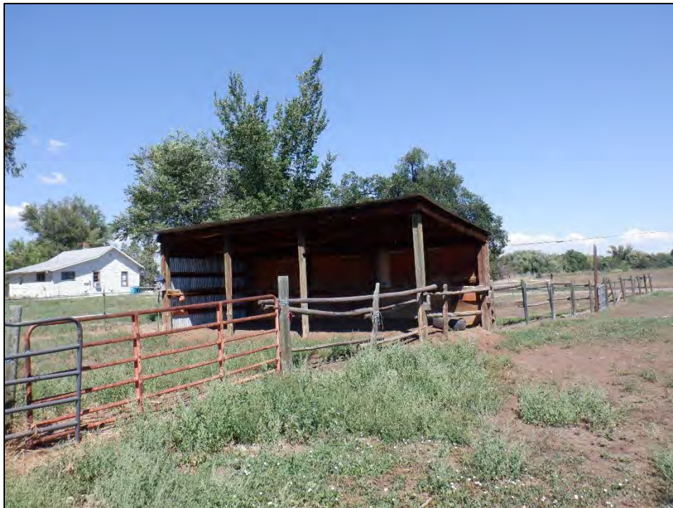
Figure 12: Feature 4, south and east elevations, view northwest (Image #652, RLS 8/23/2022).
