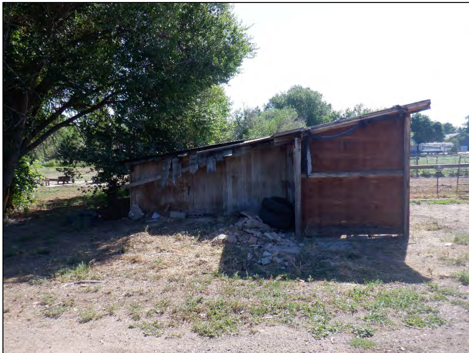
Figure 10: Feature 2, west elevation, view east (Image #600, RLS 8/23/2022).
