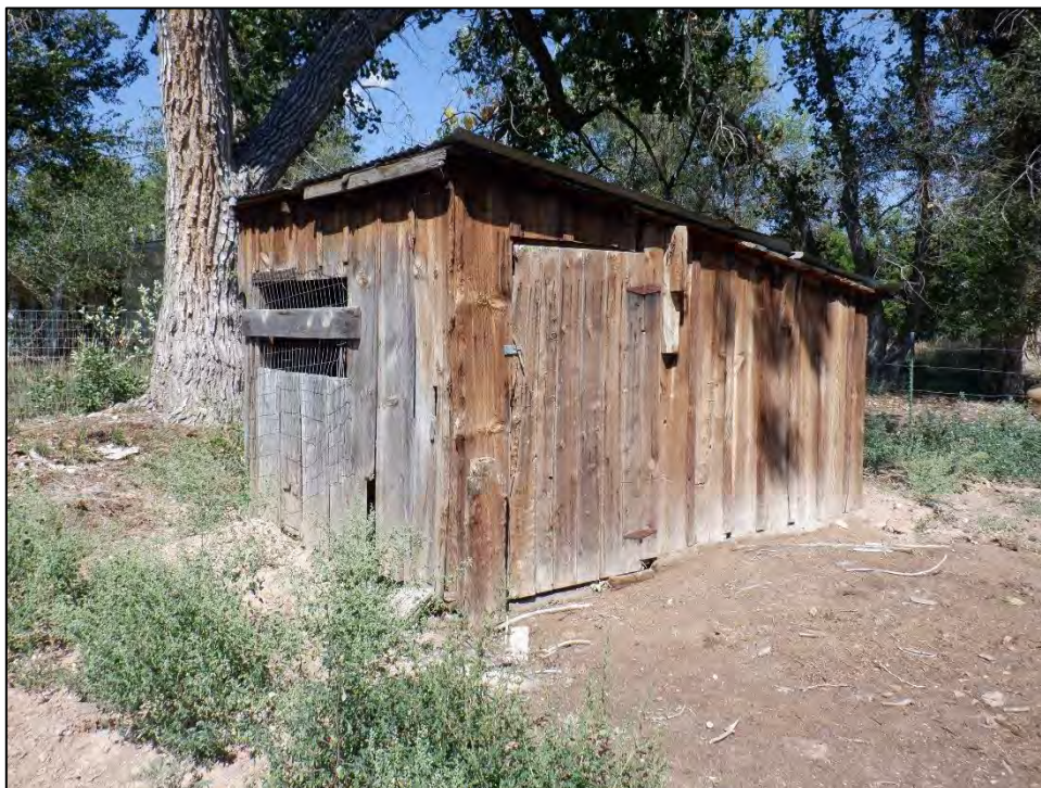
Figure 7: Feature 2, south and east elevations, view northwest (Image #634, RLS 8/23/2022).
