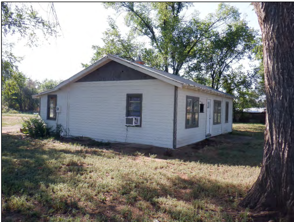
Figure 4: Feature 1, north and west elevations, view southeast (Image #581, RLS 8/23/2022).
