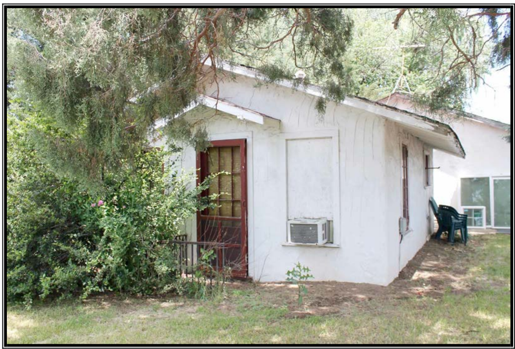
Cottage, View to the East
