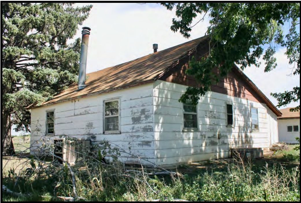
House, View to the Southeast
