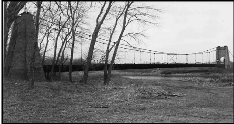
Great Western Sugar Effluent Flume
