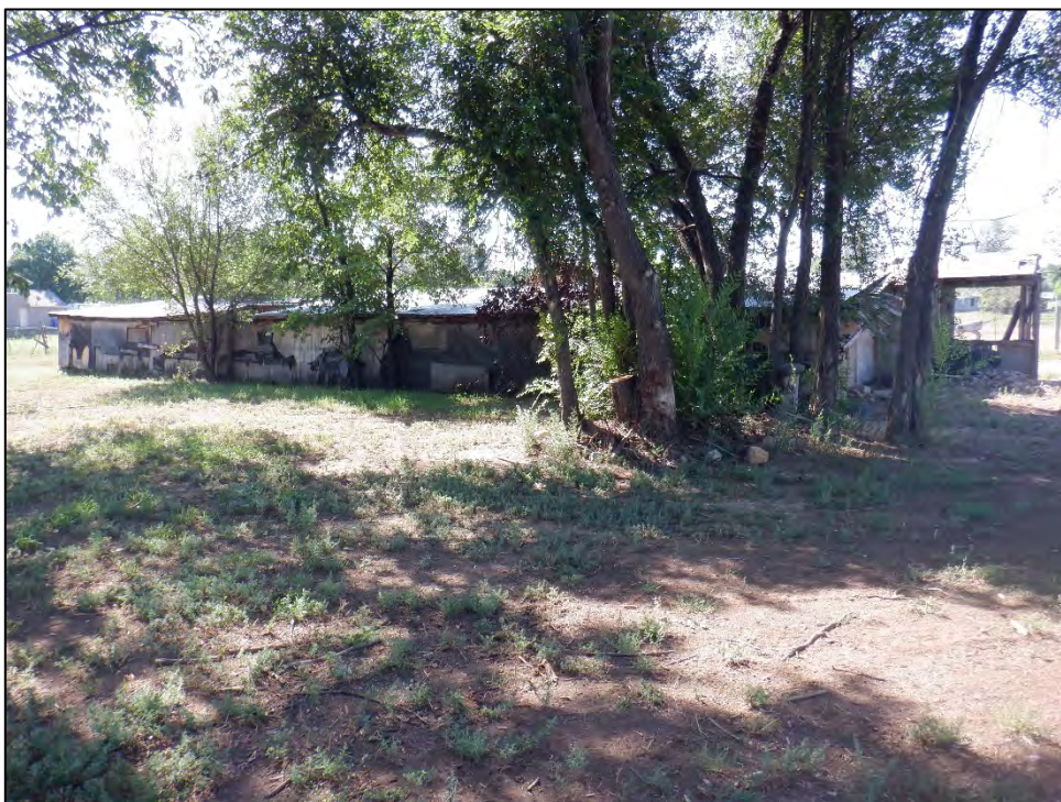
Figure 11: Feature 2, north elevation, view southeast (Image #602, RLS 8/23/2022).
