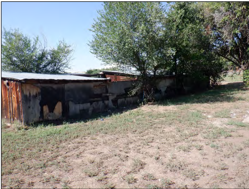
Figure 12: Feature 2, south elevation, view southwest (Image #605, RLS 8/23/2022).
