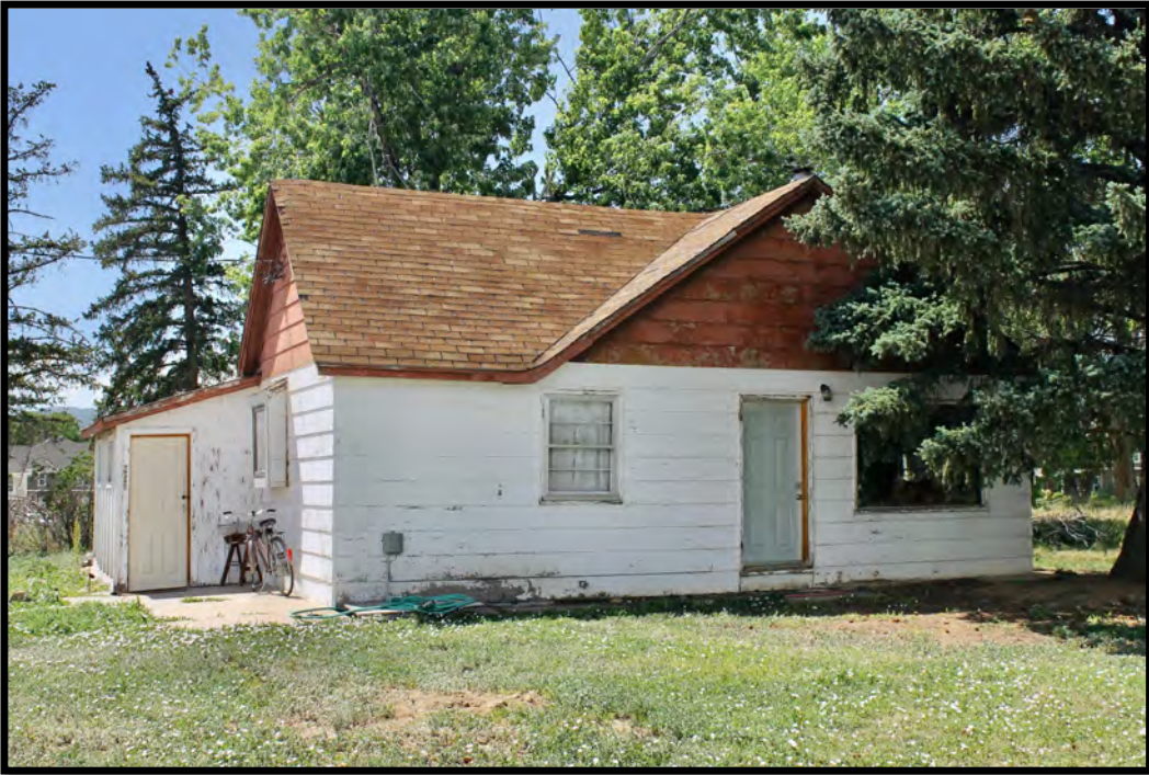
House, View to the Northwest
