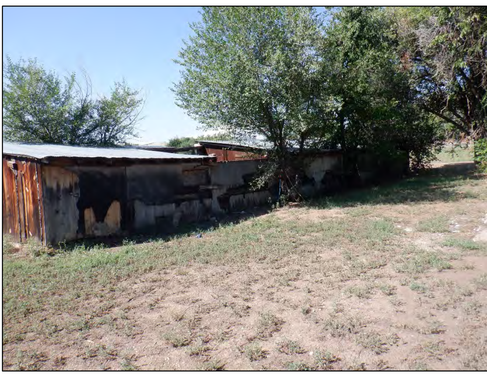
Figure 12: Feature 2, south elevation, view southwest (Image #605, RLS 8/23/2022).
