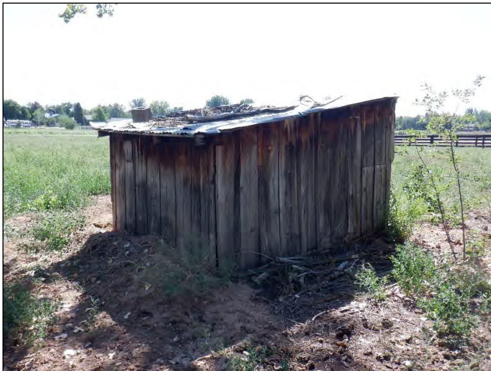
Figure 8: Feature 2, north and west elevations, view southeast (Image #345, RLS 8/23/2022).
