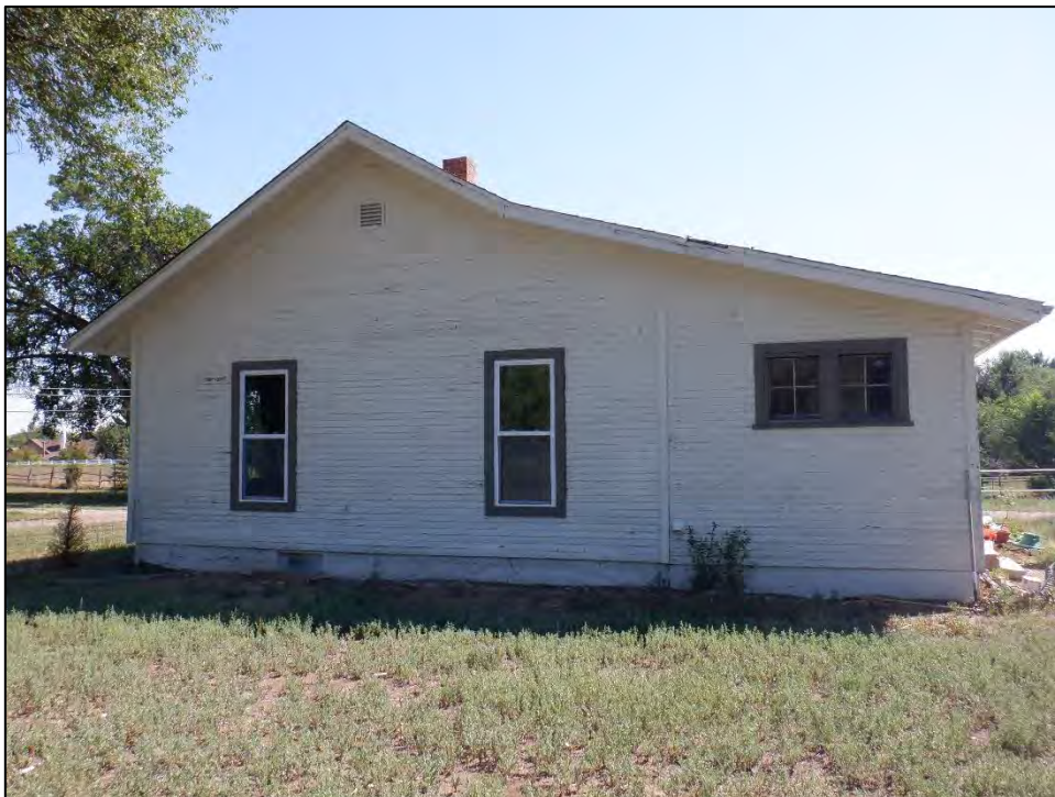
Figure 6: Feature 1, west elevation, view east (Image #639, RLS 8/23/2022).
