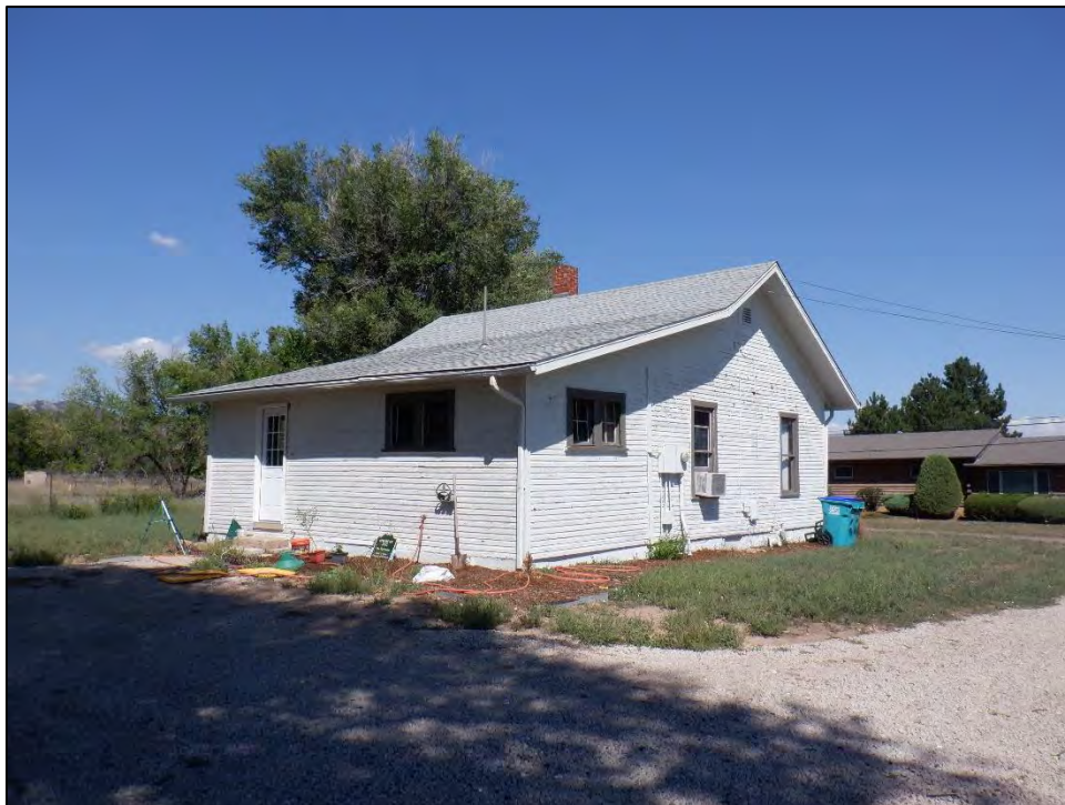
Figure 4: Feature 1, south and east elevations, view northwest (Image #637, RLS 8/23/2022).
