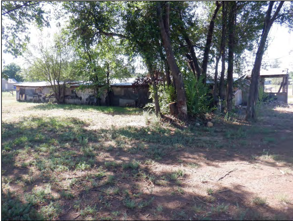
Figure 11: Feature 2, north elevation, view southeast (Image #602, RLS 8/23/2022).
