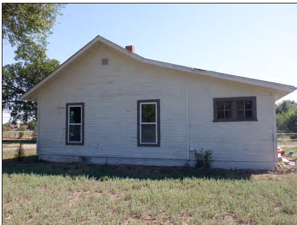
Figure 6: Feature 1, west elevation, view east (Image #639, RLS 8/23/2022).
