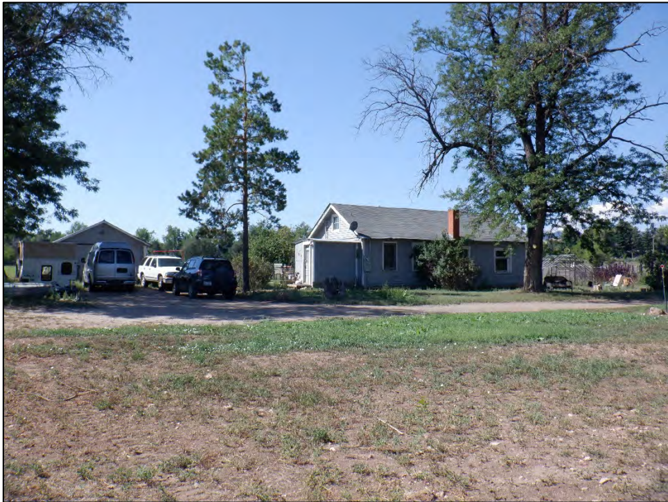
Figure 1: Site overview, view southwest (Image #632, RLS 8/23/2022).
