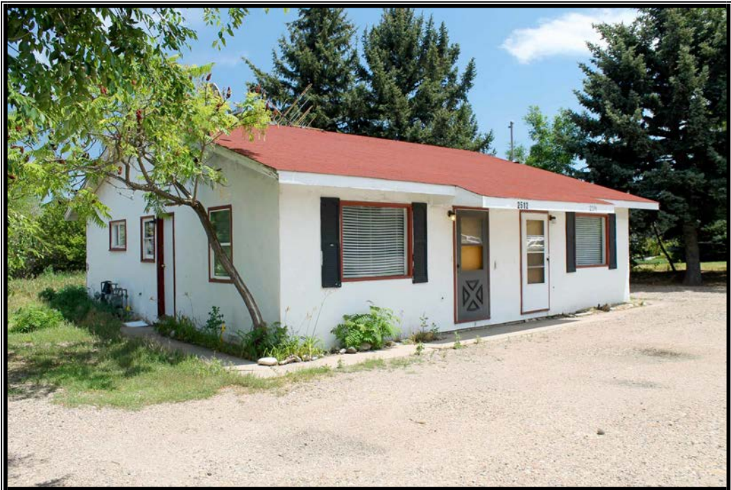
South Duplex, 2512-2514 S. Shields St., View to the Southeast
